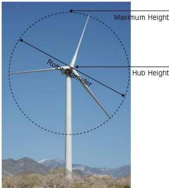
**Figure 4. Wind Turbine Features**
