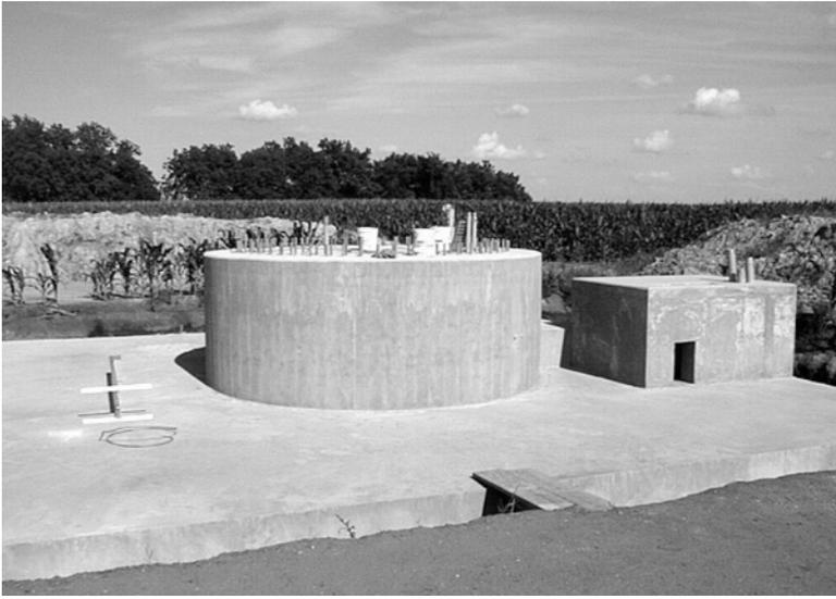
Figure 7. Inverted “T” Slab Foundation
