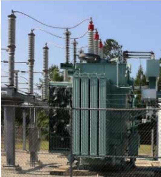
Two Winding Three Phase Transformer
