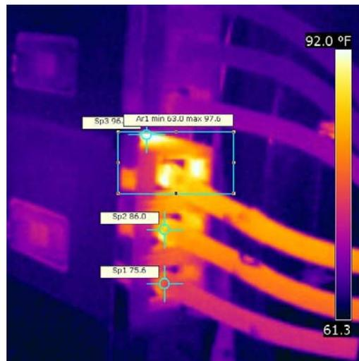
**Fig 5 – Temperature Differences between Three Sockets**
