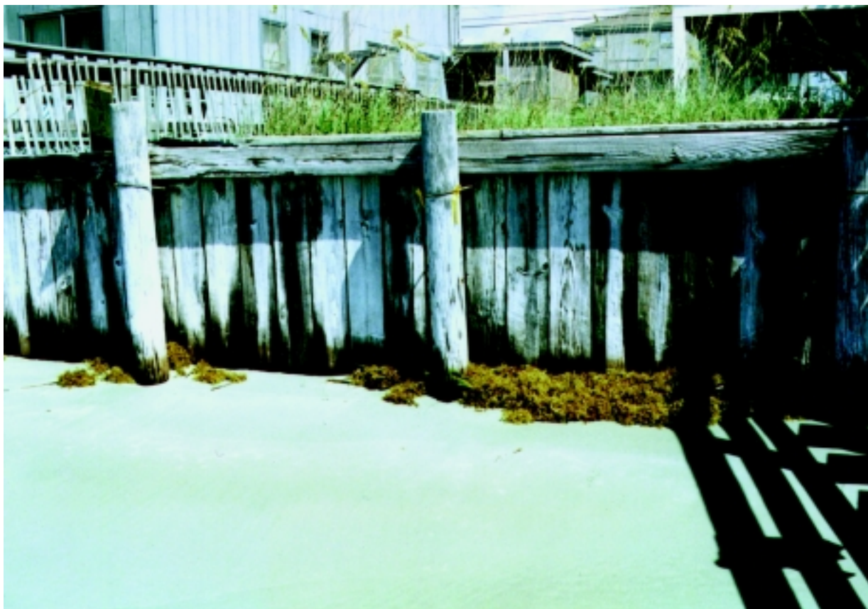
Figure 16-46 Timber bulkhead system
