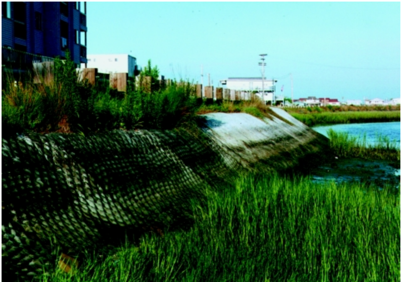
Figure 16–50 Concrete revetment (poured in place)
