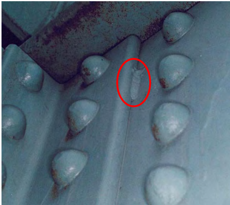
Figure 65. Photo. Tack weld used to temporarily hold a connection angle in place prior to riveting.
