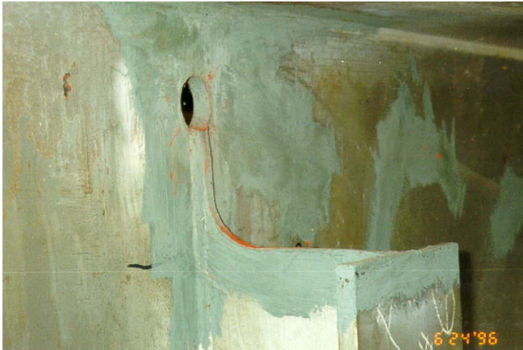
Figure 45. Photo. Web softening technique of Lexington Avenue Bridge. Photo courtesy of Minnesota Department of Transportation.
