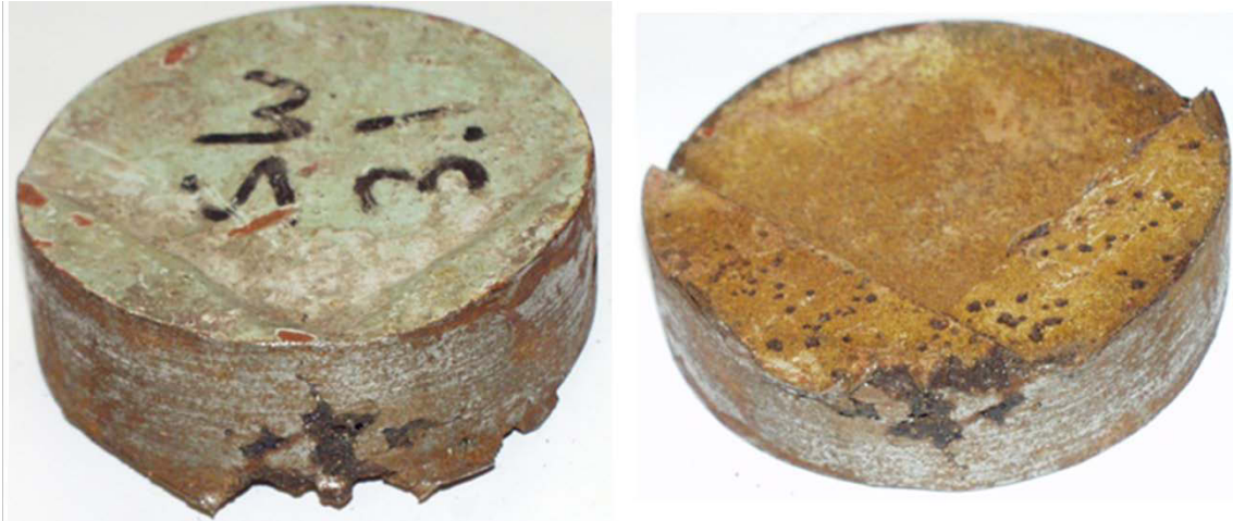
Figure 72. Photo. Core taken from intersecting welds between gusset plate, girder web, and connection plate. View of top of the gusset (left) and bottom of the gusset (right). Cores courtesy of Wiss, Janney, Elstner Associates.
