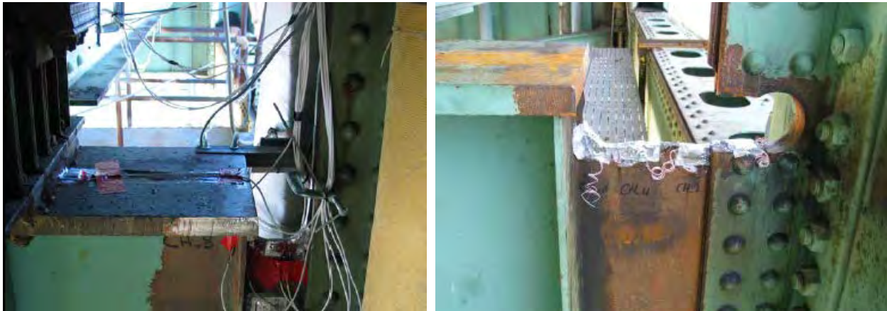
Figure 53. Photo. First retrofit performed on Girard Point Bridge in Philadelphia, Pennsylvania (left) and modified retrofit (right). Taken from Mahmoud and Connor. (88)
