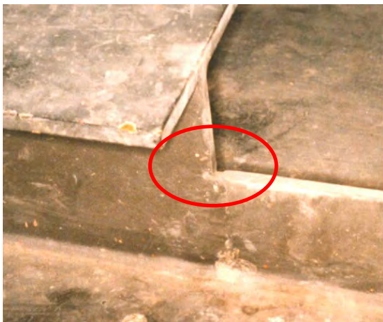
Figure 85. Photo. Bad coped beam detail with a sharp corner (left) and better coped detail with a smooth ground transition radius (right).
