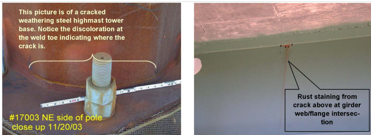
Figure 7. Photo. These two pictures show how cracks can sometimes be found from discoloration or rust staining. Photo courtesy of the Iowa Department of Transportation.
