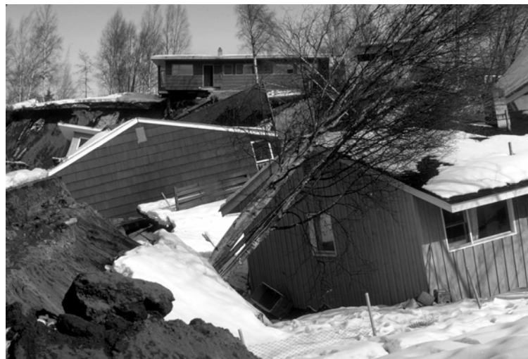
Figure 1-7 Houses damaged due to a landslide at the site. Photo Courtesy National Information Service for Earthquake Engineering, University of California, Berkeley
