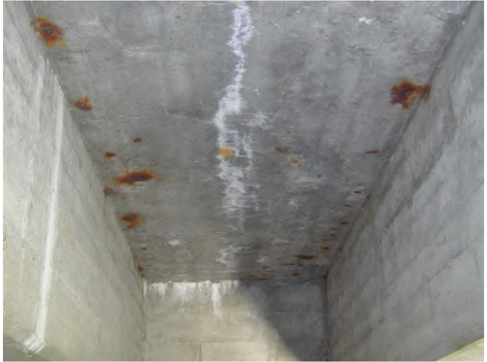
Figure 7.2.8 Underside View of Longitudinal Deck Crack
