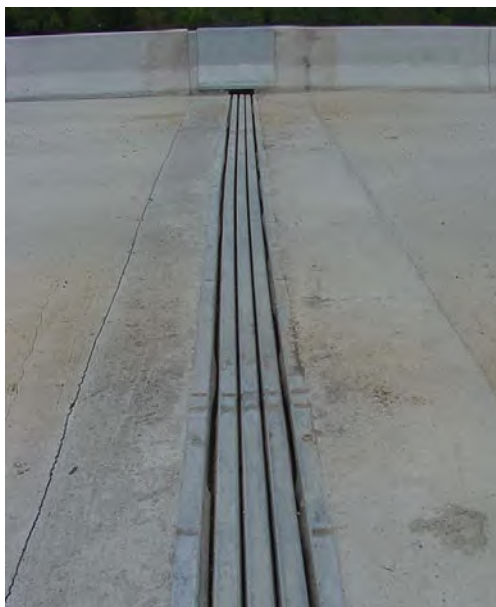
Figure 7.5.7 Modular Seal
