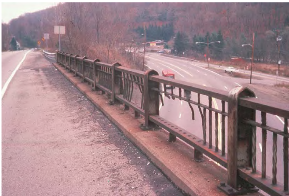
Figure 7.6.12 Deficiency Steel Post Bridge Railing
