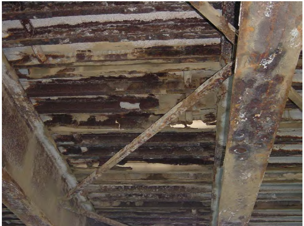
Figure 7.2.9 Deteriorated Stay-in-Place Form
