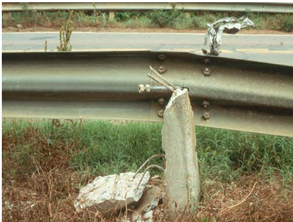
Figure 7.6.13 Approach Guardrail Collision Damage
