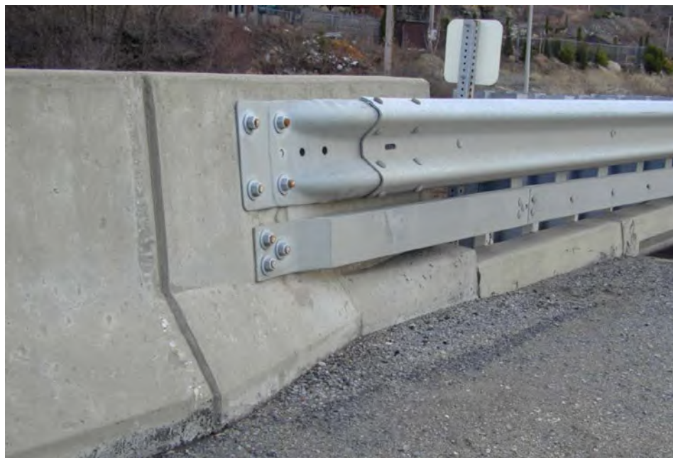
Figure 7.6.15 Proper Nesting of Guardrail at Transition
