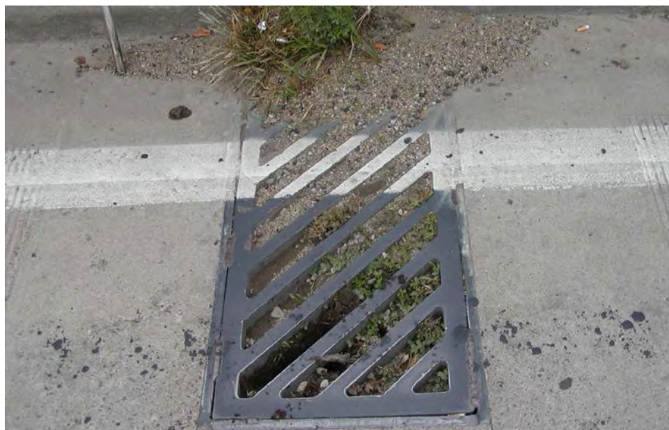
Figure 7.5.30 Clogged Scupper
