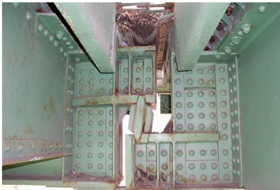
Figure 7.5.32 Drainage Trough with Debris Accumulation
