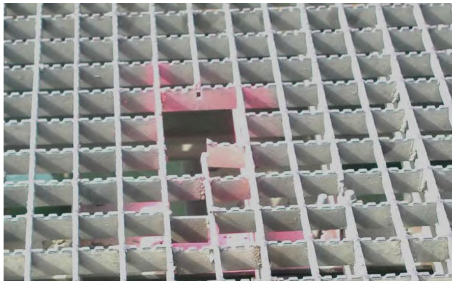
Figure 7.4.10 Broken Members of an Open Steel Grid Deck
