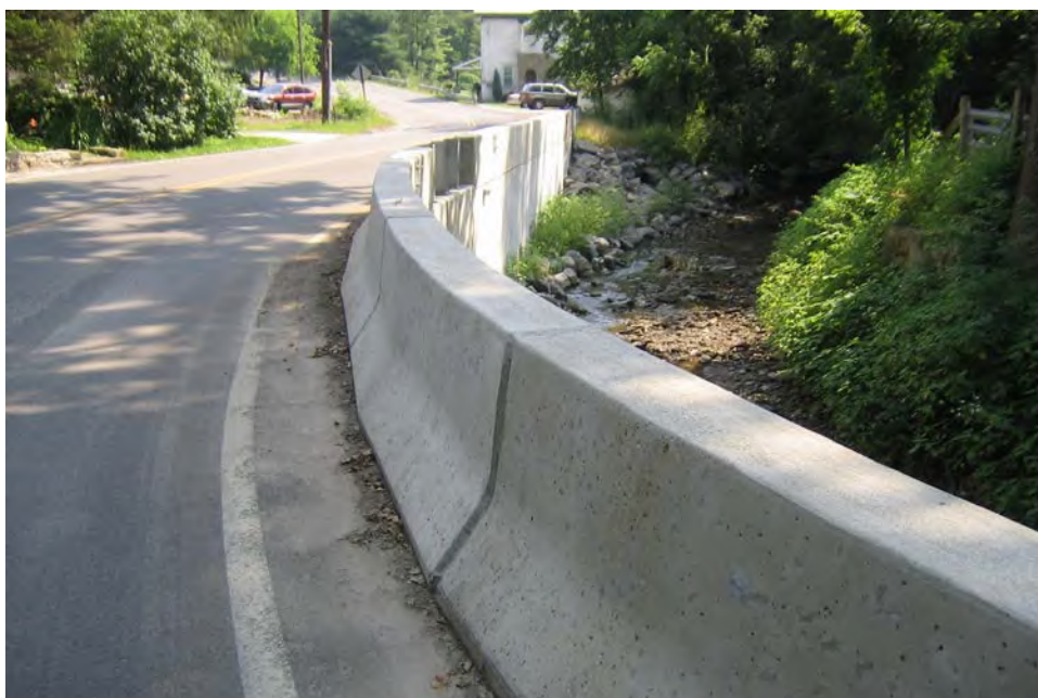
Figure 7.6.6 Acceptable Bridge Rail
