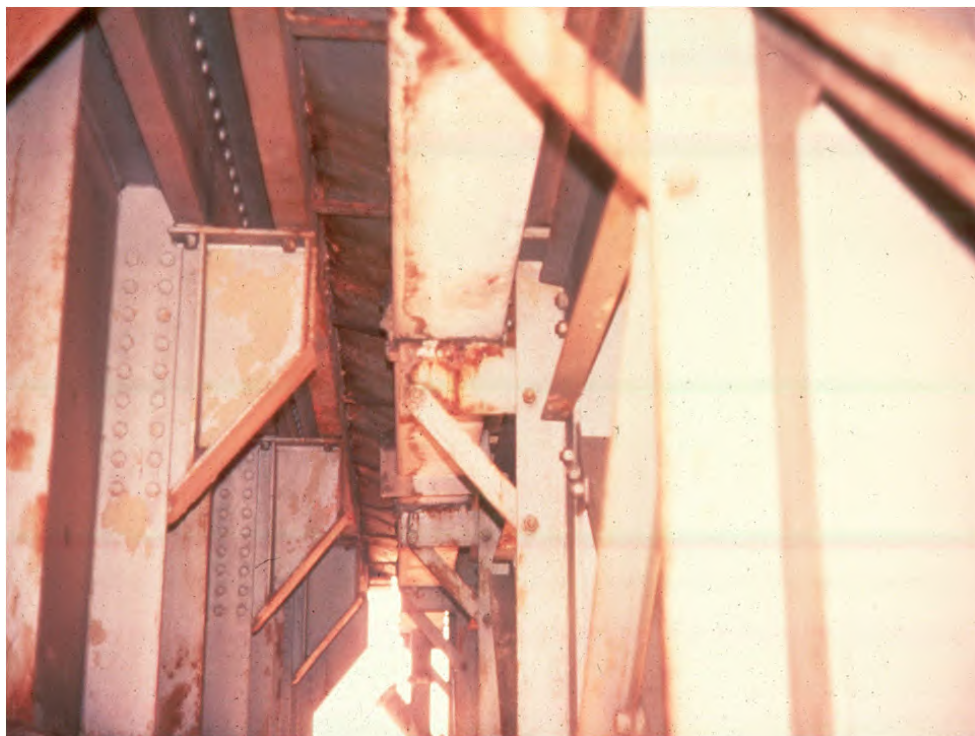
Figure 7.5.16 Supported Finger Plate Joint
