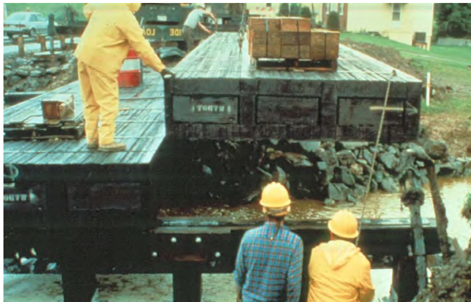
Figure 7.1.5 Structural Composite Lumber Deck Using Box Sections
