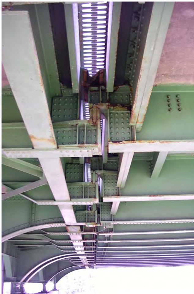
Figure 7.5.29 Support System under a Finger Plate Joint
