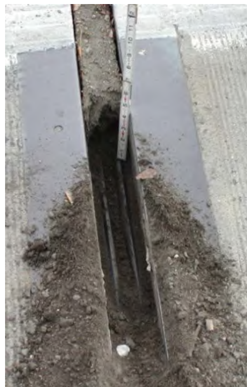
Figure 7.5.25 Dirt in a Compression Seal Joint
