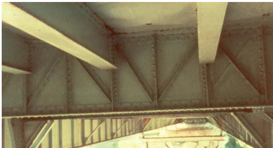
Figure 7.4.2 Underside View of Buckle Plate Deck
