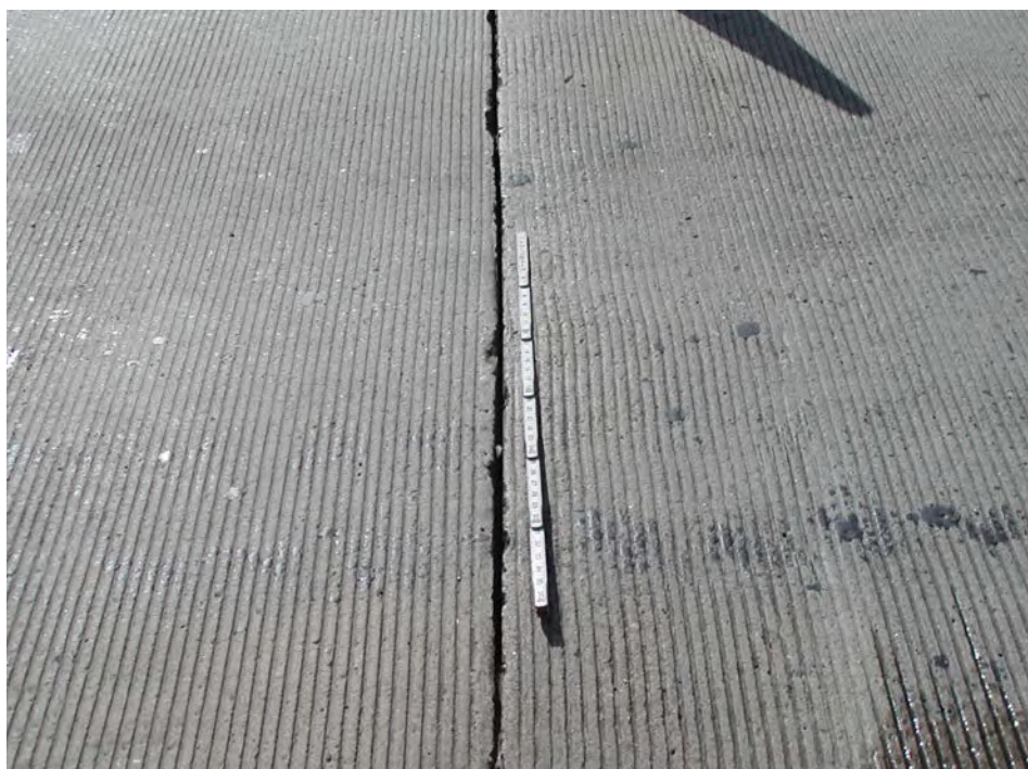
Figure 7.5.12 Open Expansion Joint
