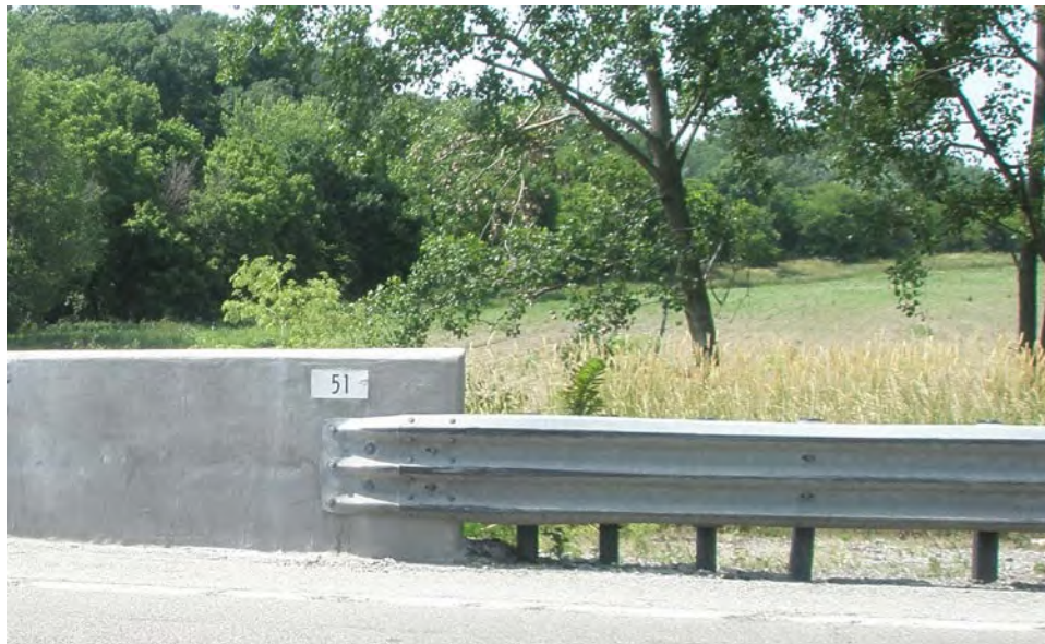
Figure 7.6.8 Acceptable Transition
