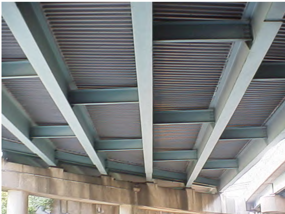
Figure 7.2.1 CIP Concrete Deck with Stay-in-Place Forms
