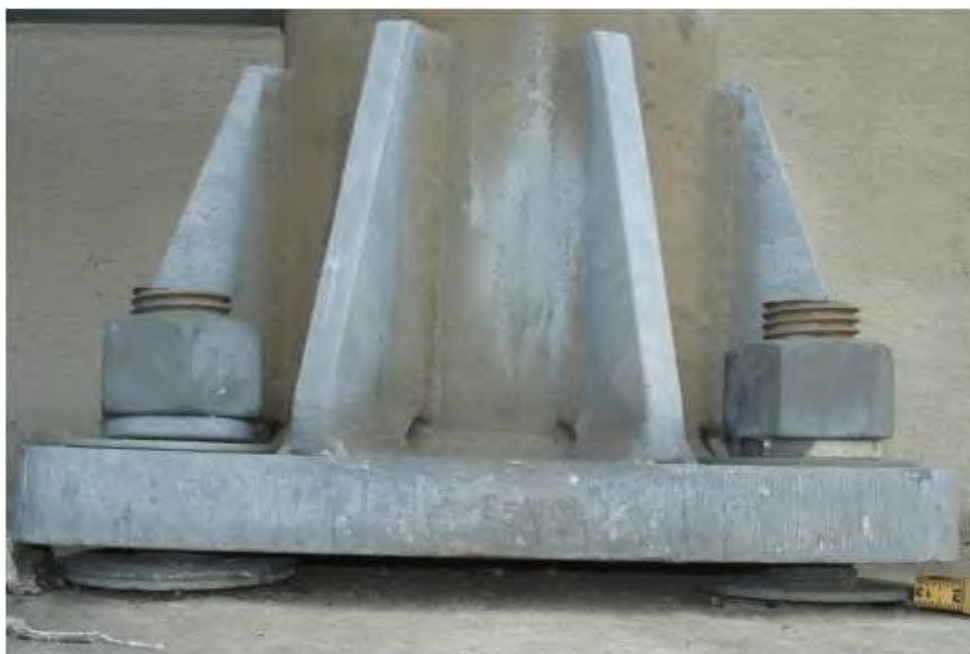
Figure 7.5.34 Sign Attachment Exhibiting Anchor Pullout
