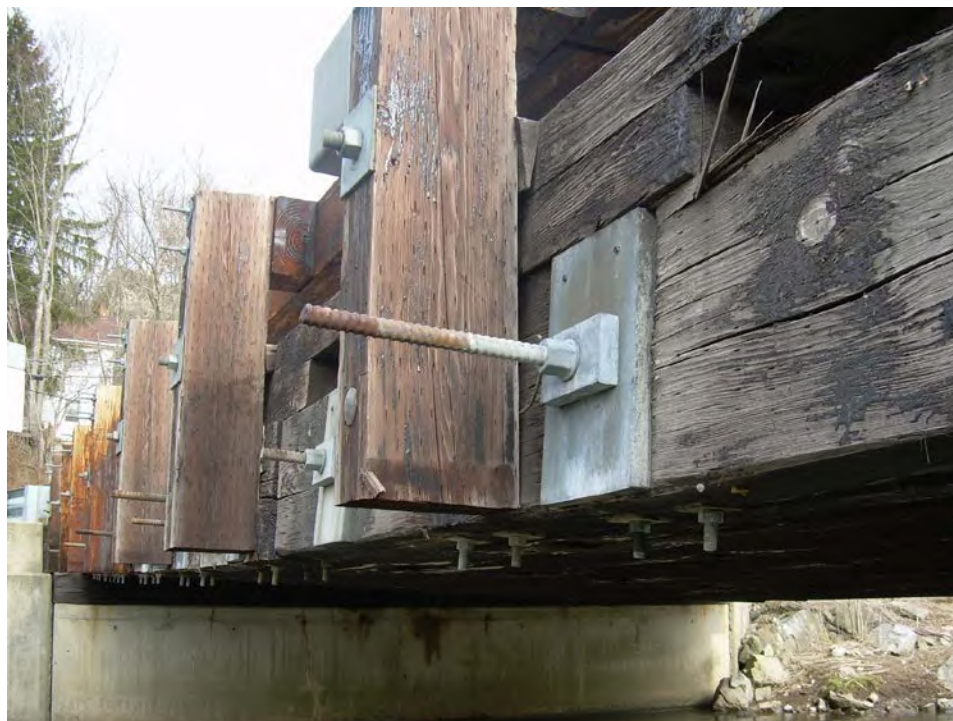
Figure 7.1.4 Stressed-laminated Deck
