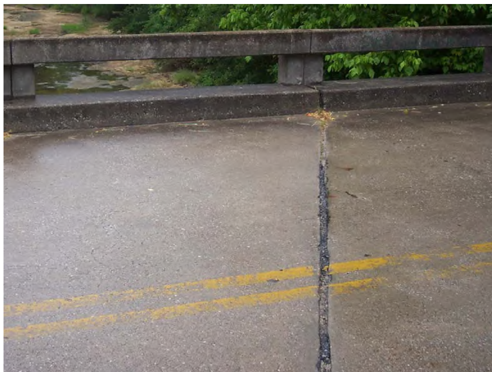
Figure 7.5.2 Pourable Joint Seal
