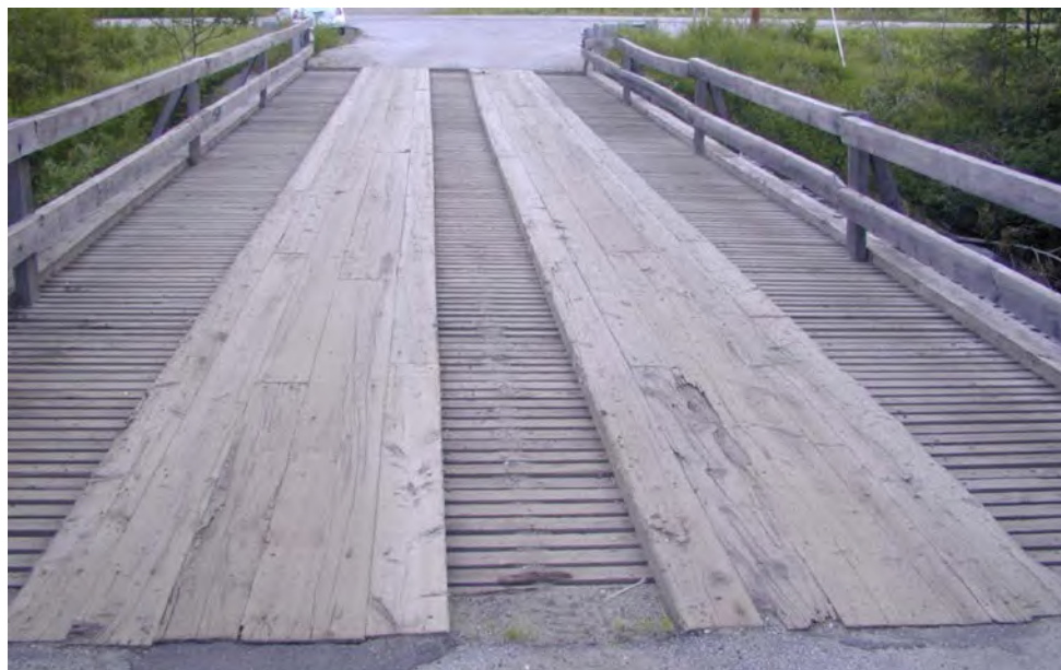
Figure 7.1.6 Timber Wearing Surface on a Timber Plank Deck
