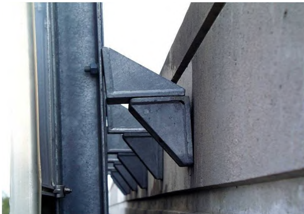
Figure 7.5.35 Sign Mount with Loose Adhesive Anchorage
