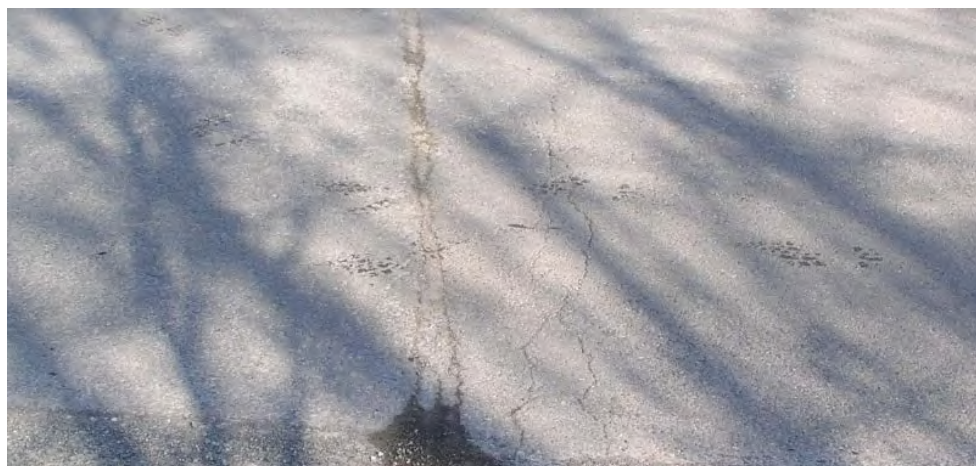
Figure 7.5.28 Asphalt Wearing Surface over an Expansion Joint
