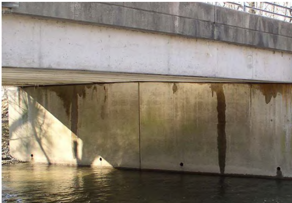
Figure 7.5.23 Weep Holes
