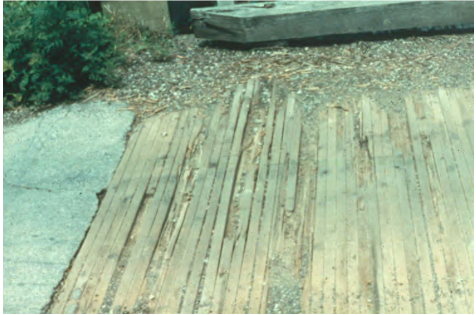
Figure 7.1.8 Wear and Weathering on a Timber Deck
