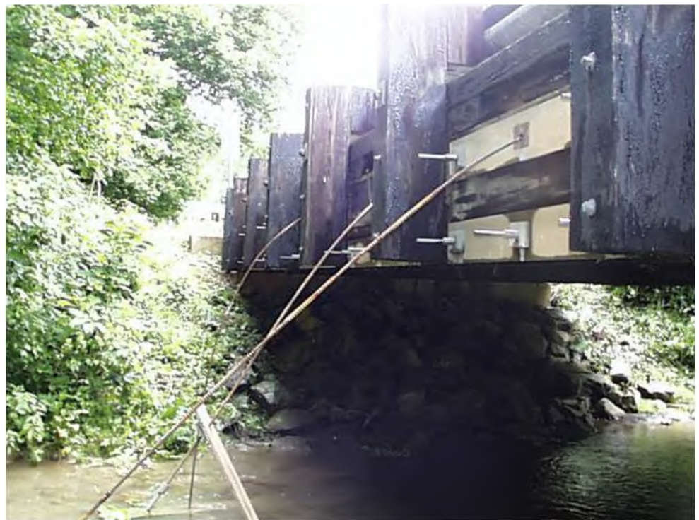
Figure 7.1.11 Broken Prestressing Anchors
