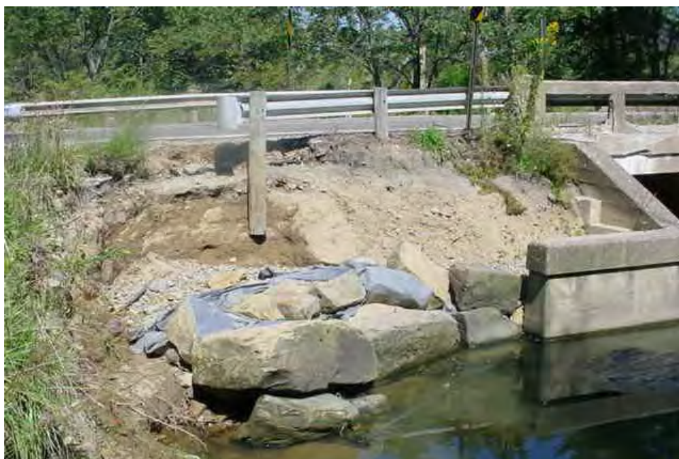
Figure 7.6.14 Erosion Reducing Post Embedment
