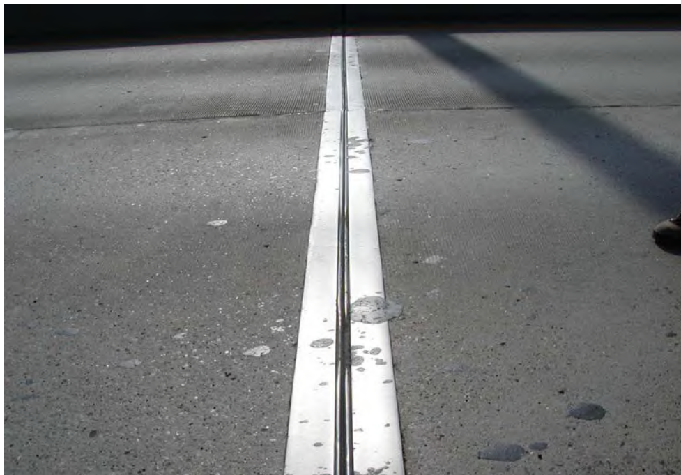
Figure 7.5.4 Compression Joint Seal with Steel Angle Armoring
