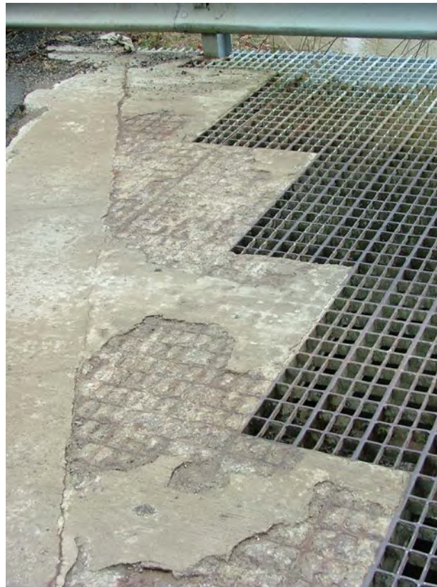
Figure 7.4.8 Filled and Un-filled Steel Grid Deck
