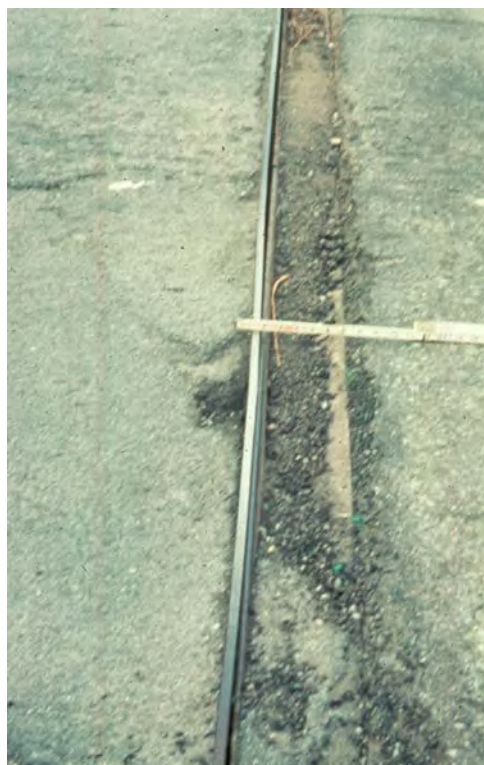
Figure 7.5.24 Debris Lodged in a Sliding Plate Joint
