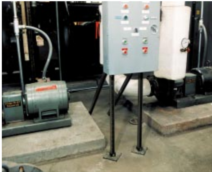
Figure 154: Typical control panel support using angles. Additional angle supports may be required (see below).
