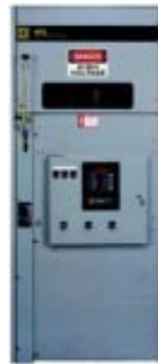
Figure 31: High voltage circuit interrupter (floor-mounted).
