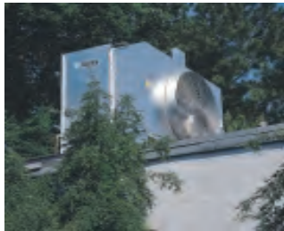
Figure 36: Fluid cooler cross flow with self-contained sump.
