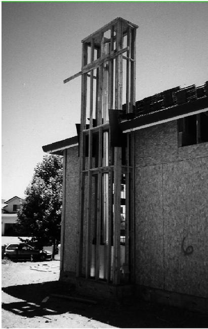
Figure 7-7 Factory-built flue and light-frame enclosure.
