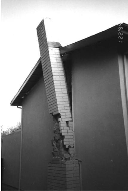
**Figure 7-2 Chimney damage in Northridge earthquake.**
