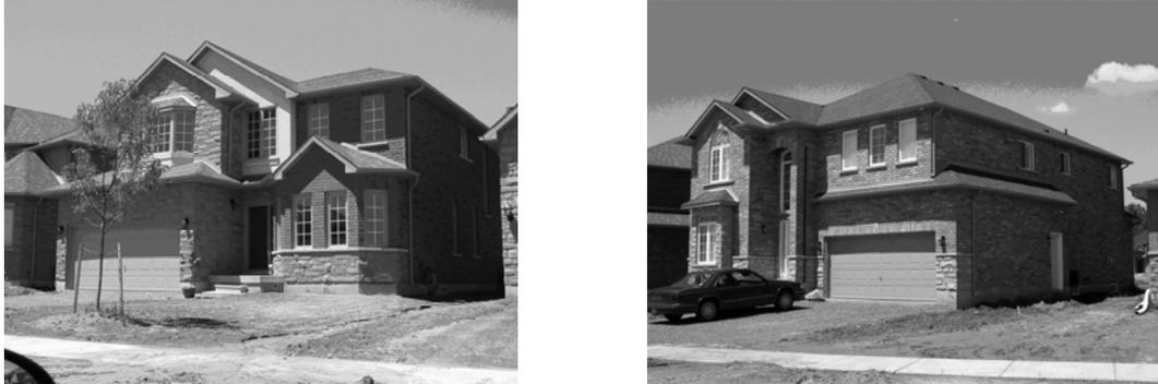
**Figure 5-11 Applications of masonry and stone veneer.**
