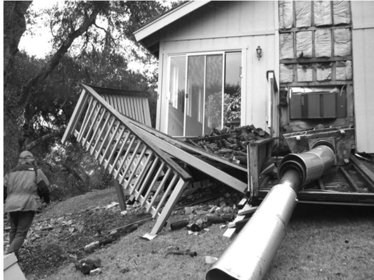
Figure 7-8 Collapsed factory-built chimney, light-frame enclosure, and deck after the San Simeon earthquake. Photo courtesy of Josh Marrow, Simpson Gumpertz and Heger Inc.
