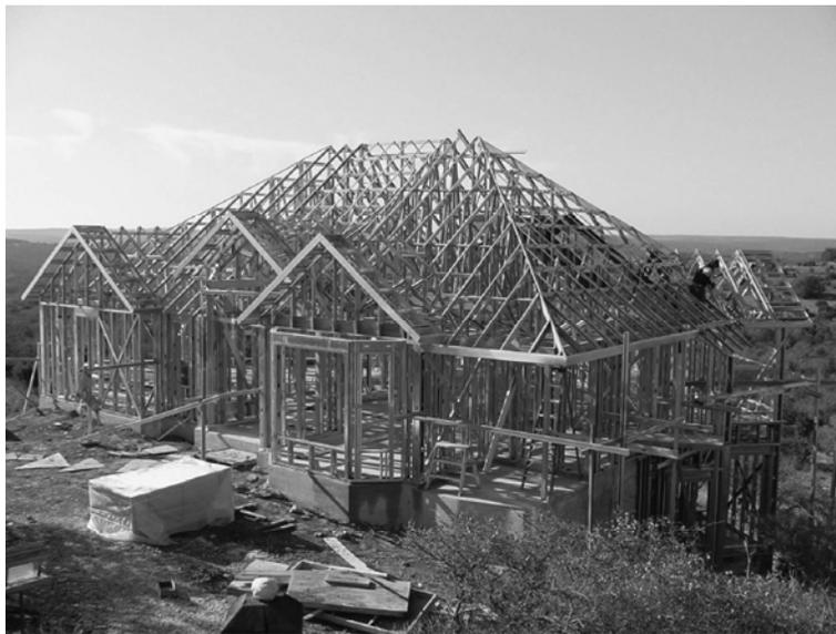
**Figure 5-13 Cold-formed steel house under construction.**
