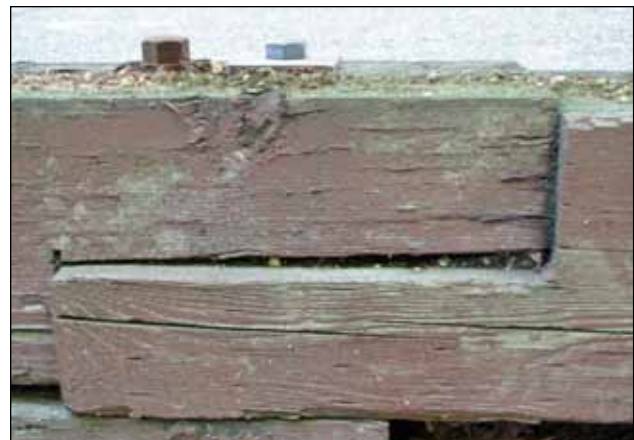
Figure 16. Unless it was pressure-treated after fabrication, this type of connection is a recipe for decay. It exposes untreated wood and creates an area that traps and holds moisture.
