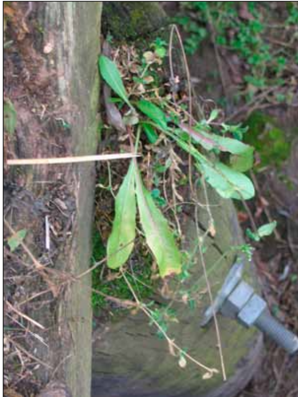
Figure 10. These piles are at risk of developing internal decay, and it is likely that the pile on the bottom already has substantial decay. Although cutting piles to height after installation is a common practice, the exposed untreated wood should be field treated and then protected with a durable cap. In this case, the tops are only partly protected, and organic matter is accumulating on the pile tops.
