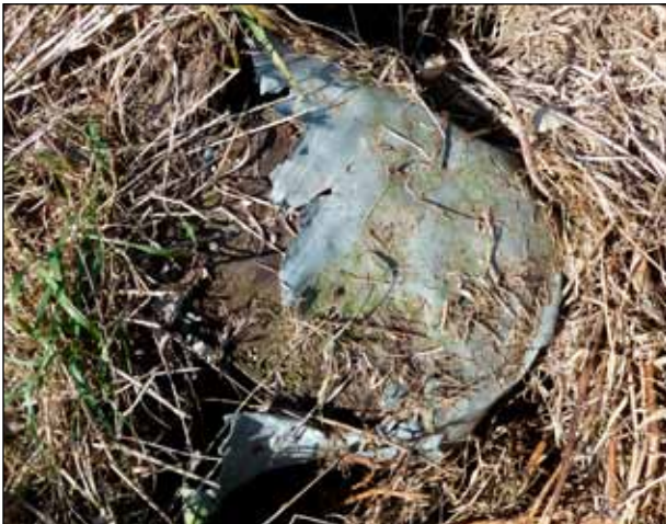
Figure 22. Galvanized pile caps (top) can provide protection of cut surfaces if applied at the time of construction. However, pile caps alone do not stop decay that has already started, and they must be inspected to ensure that they have not been damaged (bottom).
