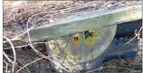
Figure 11. The older pile pictured on the bottom demonstrates how decay eventually develops in the untreated core of piles that have been cut to height on the job site. Cutting the piles at an angle with the intent of encouraging water to run off does not inhibit decay.
