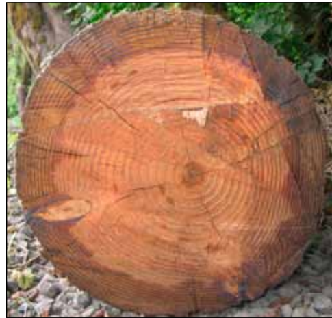
Figure 6. Vandals removed sections of cladding on this bridge, exposing the support members to moisture and decay.
