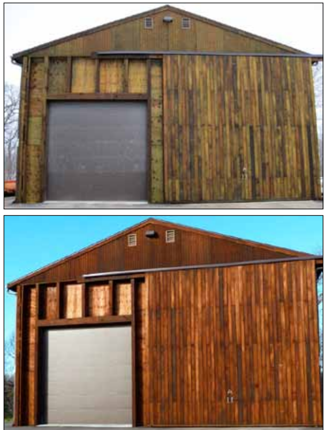
Figure 30. The green color of copper naphthenate tends to weather to brown over time. The photograph on the top is soon after construction and that on the bottom one year later. This wood was pressure-treated.
