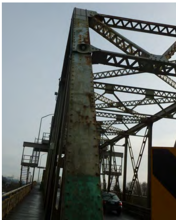
Figure 7. Southeast-bound US 101 Bridge
