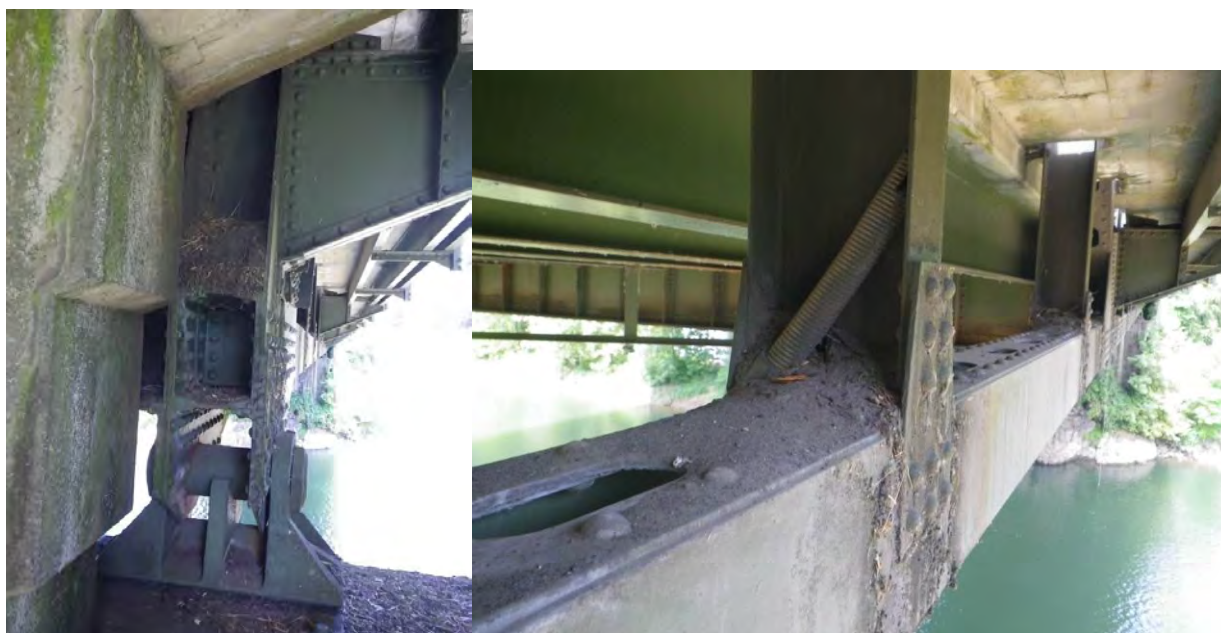
Figure 1. Bottom chord ends
