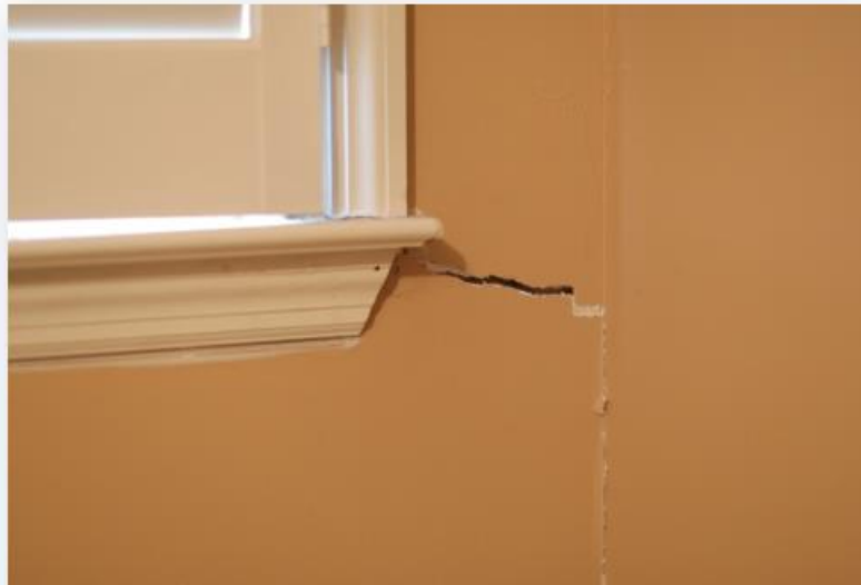
Figure 5. Drywall cracks
