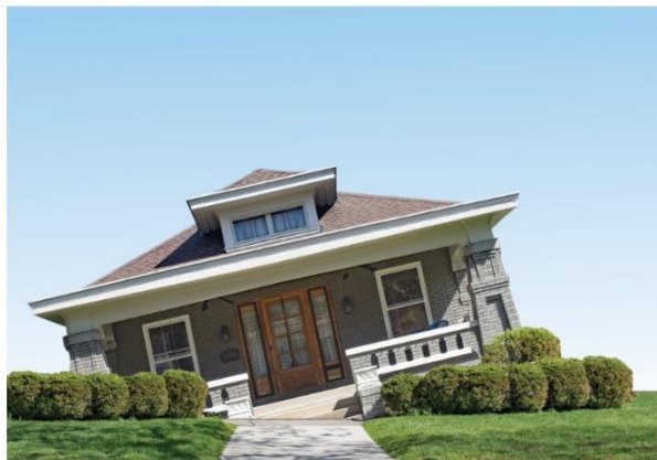
Figure 1. Differential Foundation Settlement
