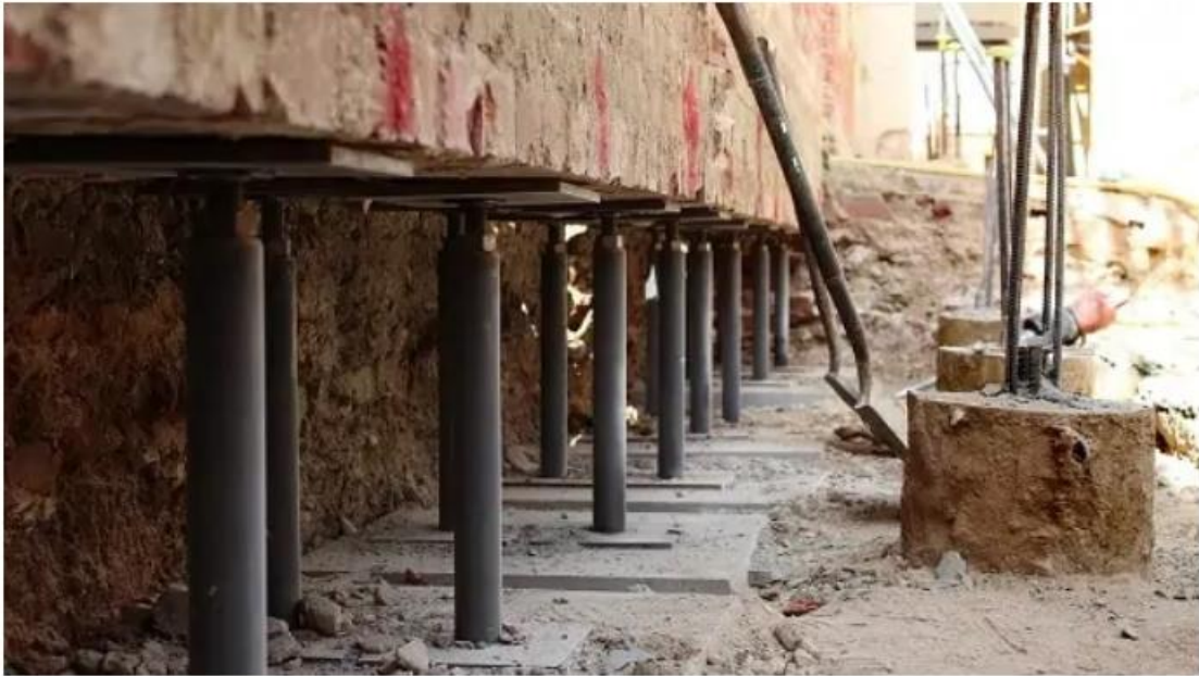
Figure 12. Underpinning
