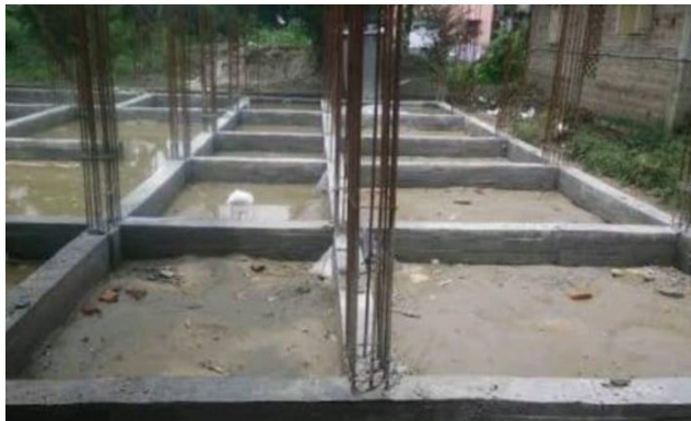
Figure 9. Tie Beams
