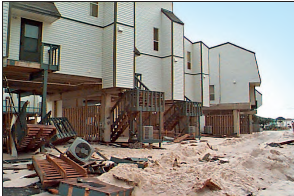
Figure 12-1. Condenser damaged as a result of insufficient elevation, Hurricane Georges (U.S. Gulf Coast, 1998)
