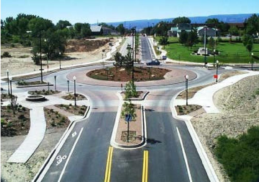
Figure 3.55– Example Pedestrian and Cyclist Treatment (Source: NCHRP 672<sup>2</sup>)
