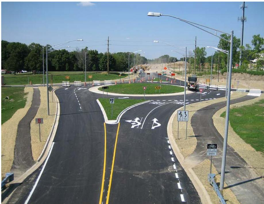
Figure 5.2 – Typical Pole Placement Plan Using Cobra-Style Luminaire
