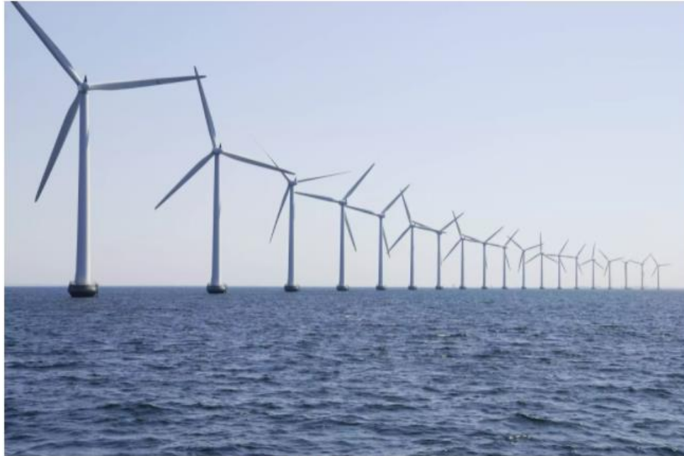
Offshore Wind Energy
