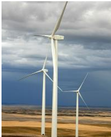
Figure 25: Land-based wind turbine
