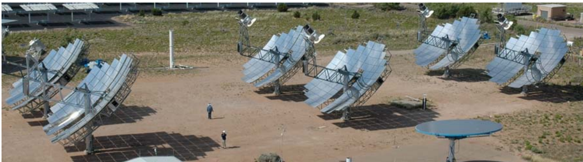
Figure 9: Prototype 150 kW dish/Stirling power plant at Sandia National Laboratory
