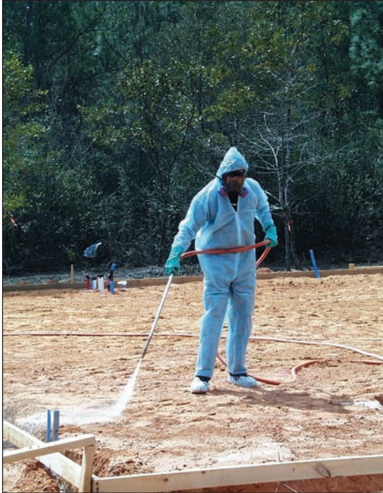
Figure 22. — Chemical treatment of fill material before slab is poured.
