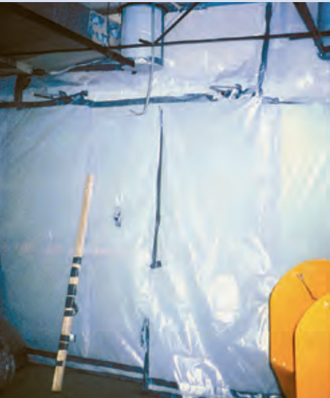
Photo 8: Full containment on large job
