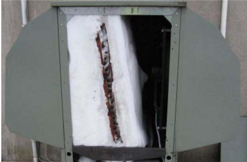
The defrost cycle can be managed with the unit's own refrigeration cycle. Here, the reversing valve switches the device to the cooling mode. This sends hot gas to the outdoor coil to melt the frost. At the same time the outdoor fan, which normally blows cold air over the coil, is shut off in order to reduce the amount of heat needed to melt the frost. While this is happening, the heat pump is cooling the air in the ductwork.
