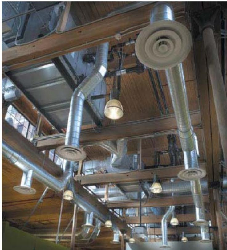
The total air flow through the geothermal heat pump/air ducting must be at the geothermal manufacturer's rated CFM (cubic feet per minute), and at the rated static pressure. If the air ducting is too small, the air will move too slowly, causing inefficient
