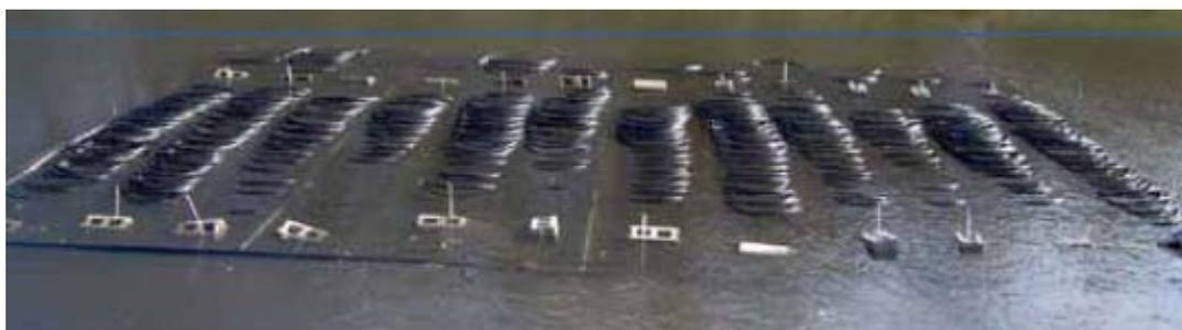
Submerged loops can be formed by coiled polyethylene pipe, mats or plate heat exchangers. Typical installations require around 300 to 500 ft. of pipe per cooling ton (27 to 45 m/kW) and approximately 3,000 ft<sup>2</sup> of surface water per cooling ton [79 m<sup>2</sup>/kW].
