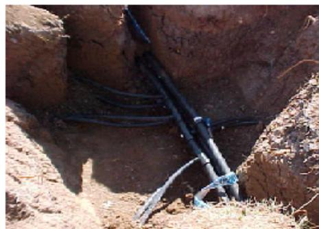
All earth loops, especially those with buried (inaccessible) fusion joints, should be pressure tested with compressed air to at least 75 psi for at least 24 hours to ensure there are absolutely no leaks.
