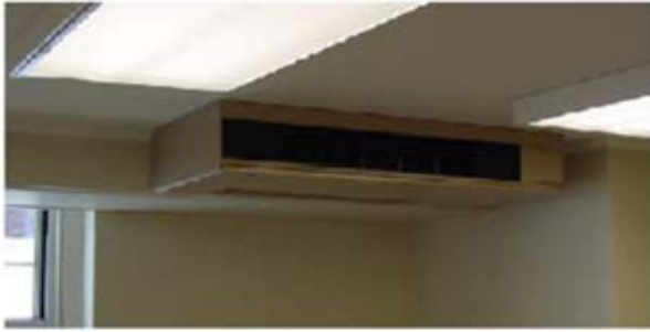
Horizontal ceiling-surface-mounted FCU
