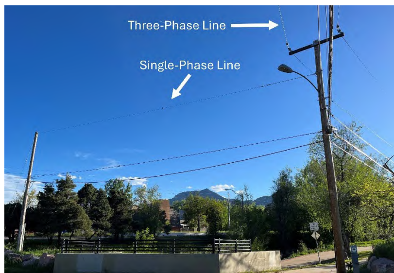
Figure 4. Annotated photo showing three-phase and single-phase distribution lines.
