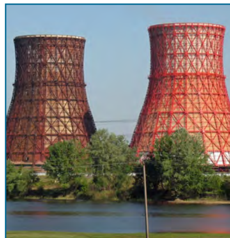
Figure 5. Hyperbolic Cooling Towers (Source: Victor Vizuz).
