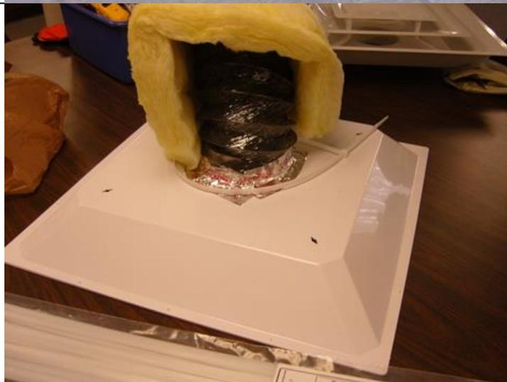
Once adjusted, tighten the zip tie and cut any excess length off. The insulation can now be pulled forward to cover the bare flex duct and zip tied again to keep it in place.
