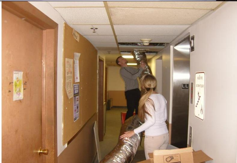
At this time, all of the flex duct will be up in the drop ceiling and all of the kinks should be worked out. If a straight run isn't possible, try to make the bends as smooth and small as possible to keep the pressure drop to a minimum.
