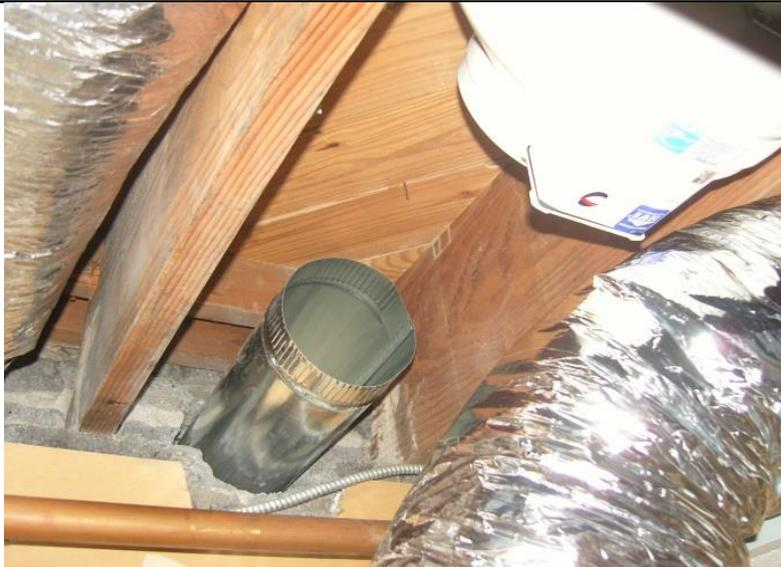
Fans can be fit between floor joints even in very tight ceilings and then mounted with the supplied bracket into the drop ceiling as well.
