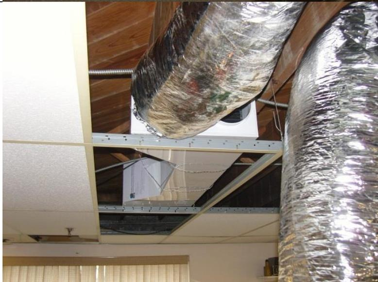
Seal the inside lining of the duct work with aluminum tape. Then secure the entire duct work with a zip tie over the insulation, aluminum tape and ERV lip the same way as connecting the duct work to the filter grill.
