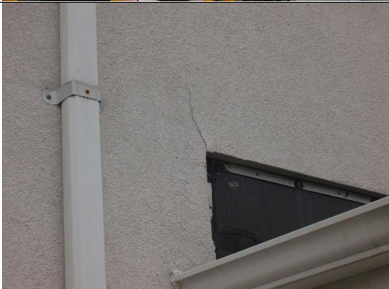
Caulk and seal the weather proof air intake exhaust to minimize water penetration issues.
