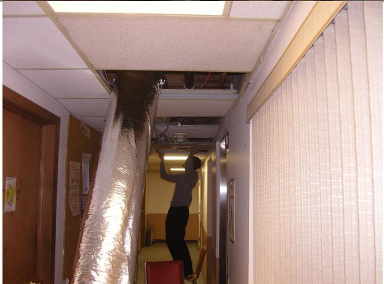
Mount the Energy Recovery Module in the drop ceiling or designated area. Most Energy Recovery Modules are difficult to install overhead and in tight spaces because of their weight and size. That is why for this application BPE-XE-MIR 200 was optimal. It is made of Polypropylene and is long and narrow.
