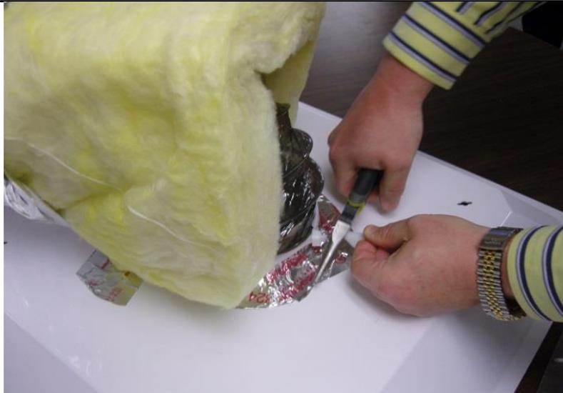
Begin installing the ductwork at the location where the exhaust grill was designed to be. Snake the opposite end from the grill up through the drop ceiling or designated area towards the ERM.
