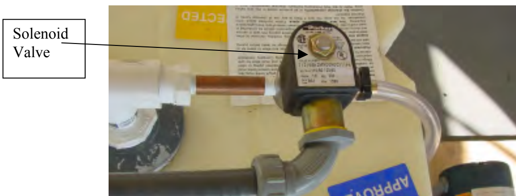
Figure 3: Normally closed solenoid valve
