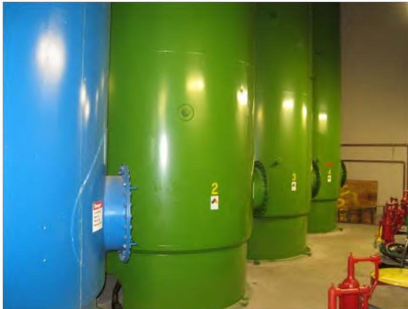
Figure 8-1. Hydroelectric Plant Turbine Oil Storage Tanks.
