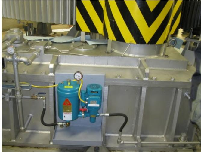
Figure 6-4. Kidney Filter for a Gearbox.
