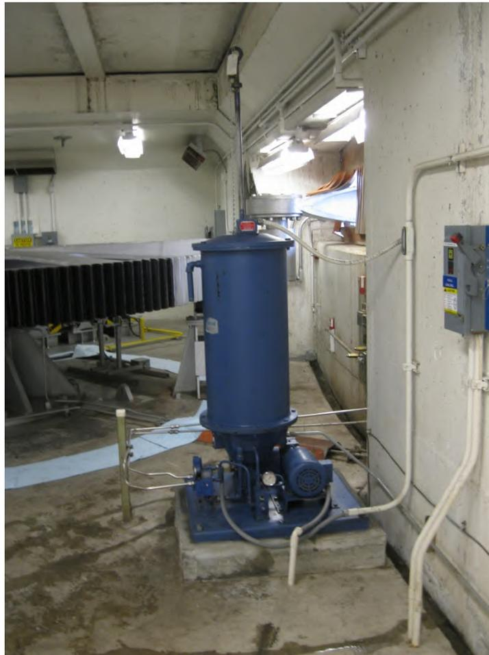
Figure 8-3. Automatic Grease-Dispensing System for Lock Machinery and Miter Gate Pintle
