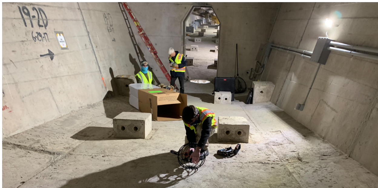
Figure 4. Workers Deploying UAS in Bridge Deck Interior (Image Courtesy: NCDOT)
