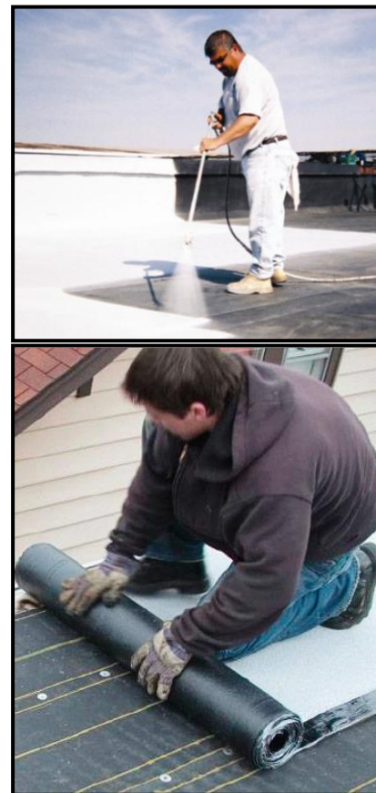
Figure 6: Two Cool Roof Installations
