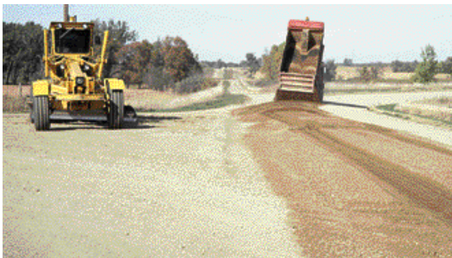
These two photos depict a the good job of spreading done by a county highway department using tandem end-dump trucks. The skill of the drivers makes this job look easy. Notice also the grader is ready to begin processing the material.
