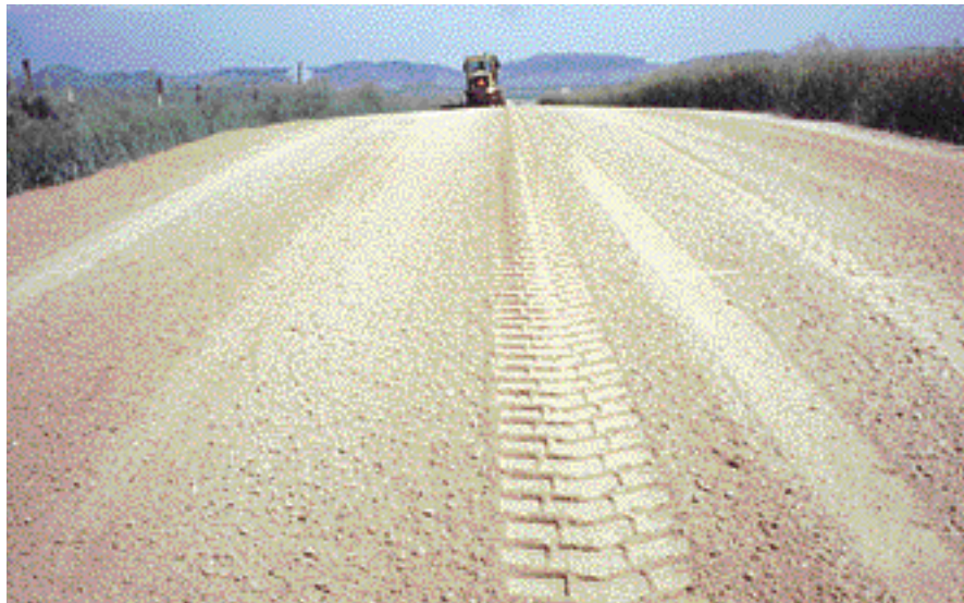
This road has been prepared well for a liquid Magnesium Chloride treatment. Notice the uniform, loose and nicely crowned surface looking over the hilltop. There is also good shoulder drainage as well. This is an excellent example of road preparation.
