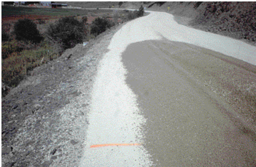
These two photos depict a the good job of spreading done by a county highway department using tandem end-dump trucks. The skill of the drivers makes this job look easy. Notice also the grader is ready to begin processing the material.
