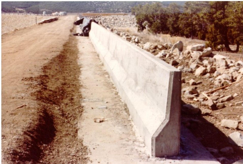
Figure F-2. Example 2: a conventional parapet wall
