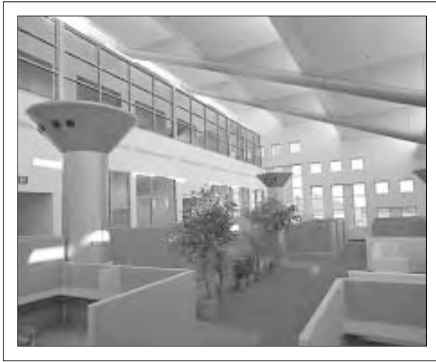
Each innovative “air tree” above provides ventilation for six offices at the National Renewable Energy Laboratory’s (NREL’s) Solar Energy Research Facility in Golden, Colorado. Air is cooled and humidified by direct evaporation, or “swamp cooling.”
