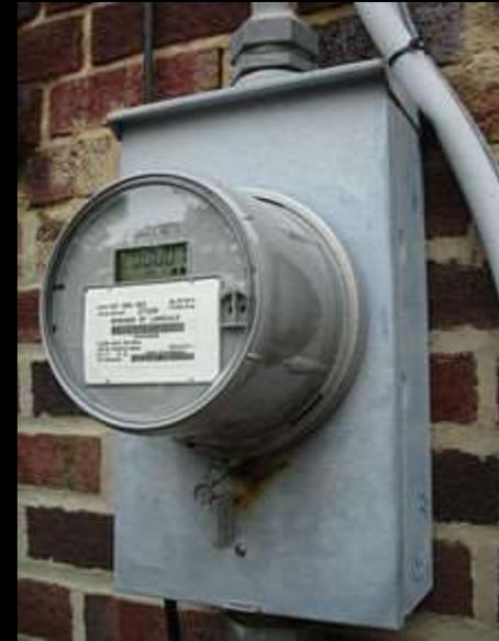
Advanced Metering Infrastructure (AMI) differs from Automatic Meter Reading (AMR) in that it has two-way communication between the meter and the power supplier.
