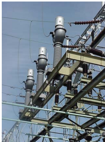
Fig. 18. Free Standing 138 kV 2000/5 A CTs
