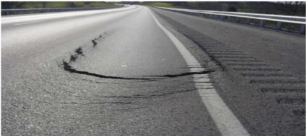
*Figure 40 Slippage Cracking*
