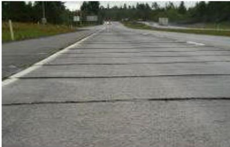
*Figure 69 Faulting from Ground Level*
