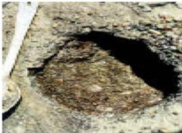
*Figure 42 Stripping at the Bottom of the Hole*
