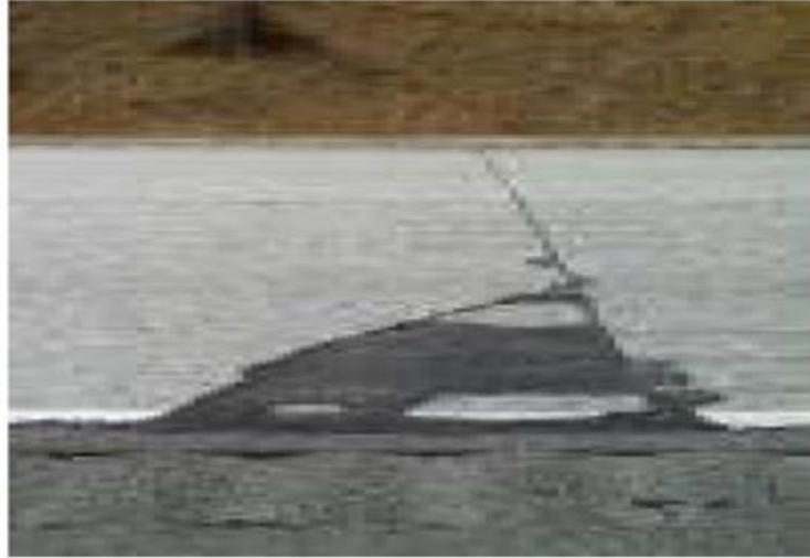
*Figure 72 Patched Failure*
