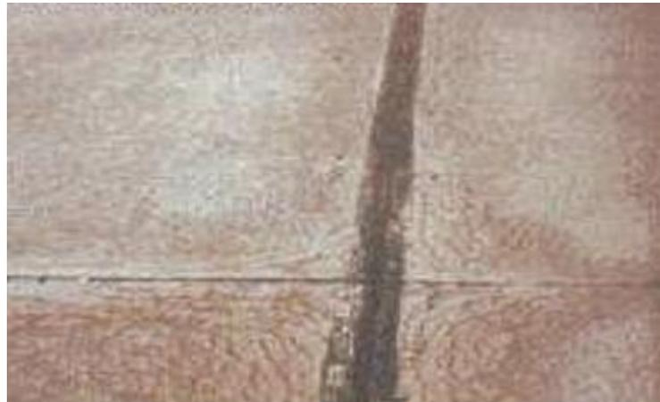
*Figure 68 D Cracking at Panel Corners*
