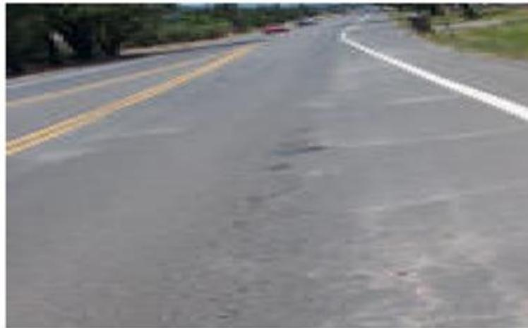
*Figure 48 Cement Treated Base Pumping through HMA Cracks*
