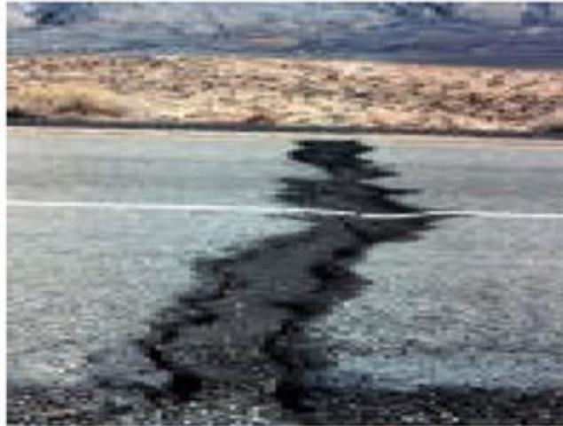
*Figure 44 Large Patched Thermal Crack*
