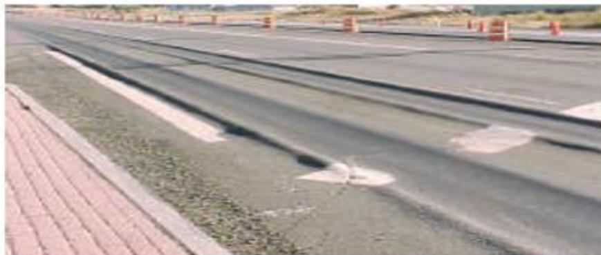
*Figure 39 Rutting from Mix Instability*
