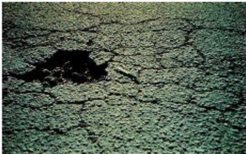
*Figure 36 Pothole from Fatigue Cracking*
