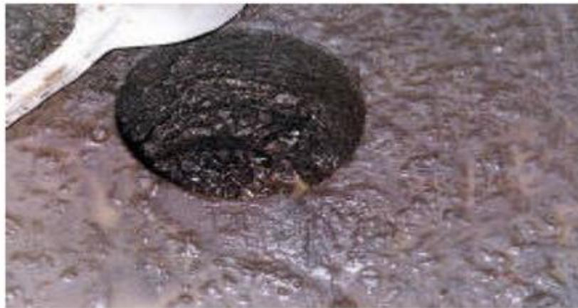
*Figure 41 Core Hole showing Stripping at the Bottom*
