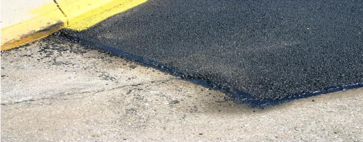
*Figure 51 New Asphalt Binder over an Existing Pavement*
