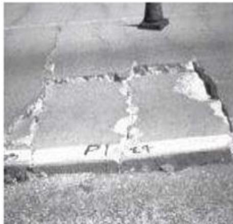
*Figure 86 Severe Punchout*
