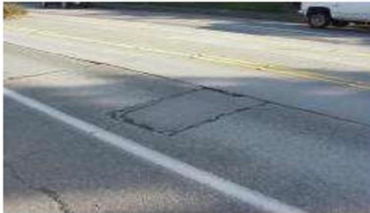
*Figure 77 Patching with Poor Edges*
