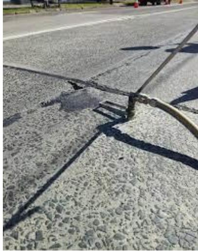
*Figure 93 Slab Jacking*
