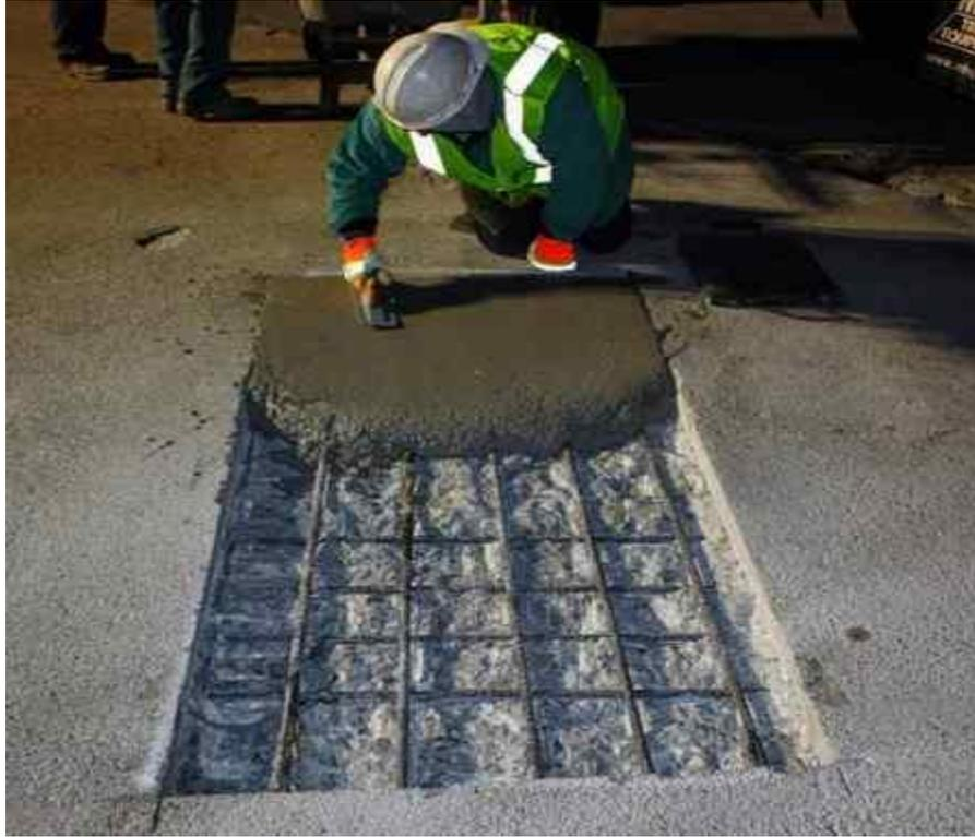
*Figure 94 Partial Depth Repair*
