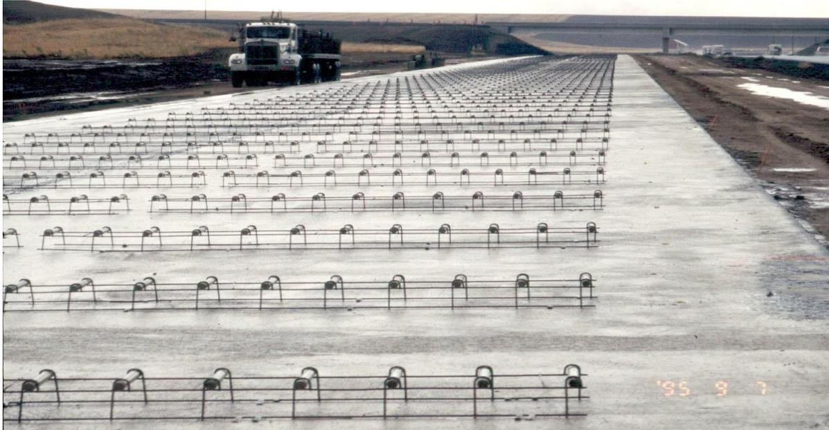
*Figure 17 Dowel Bars in Rigid Pavements*
