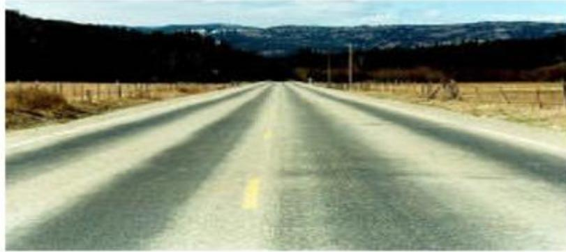
*Figure 22 Bituminous Surface Treatment Bleeding in Wheel Paths*
