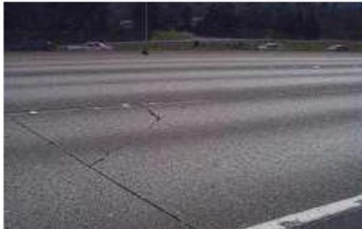
*Figure 67 Corner Break on a Highway*
