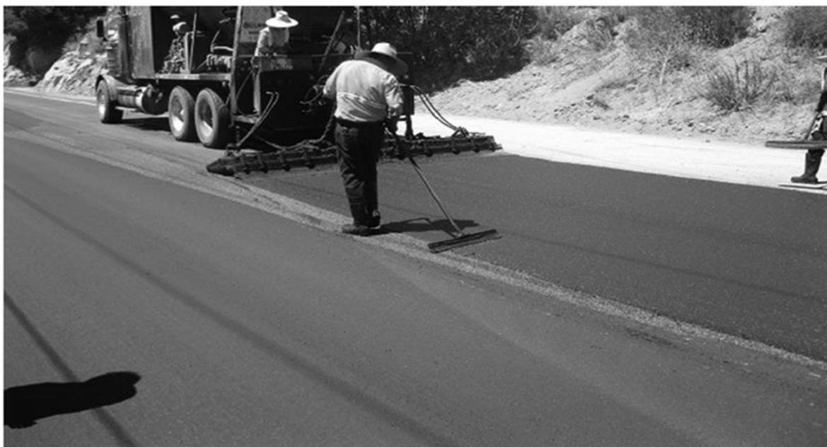
*Figure 58 Microsurfacing*
