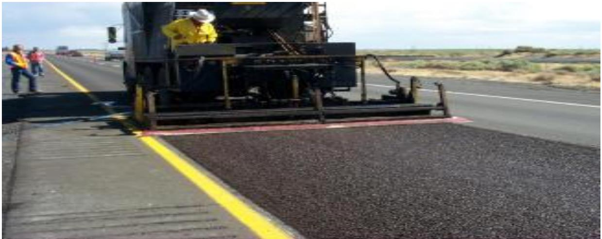
*Figure 55 Slurry Seal Application*
