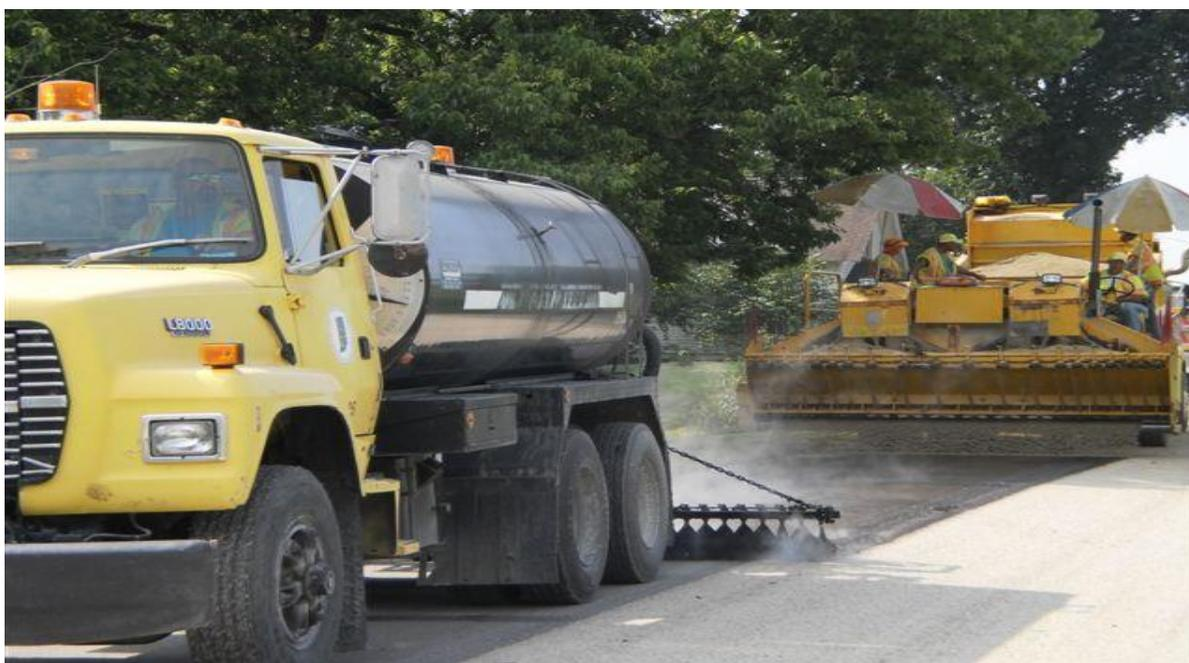
*Figure 57 Chip Seal Application*
