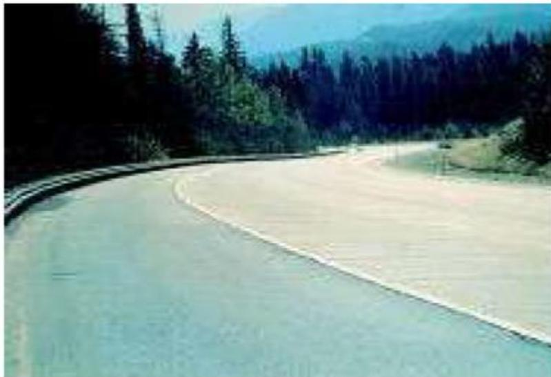
*Figure 70 Faulting in the Truck Lane*
