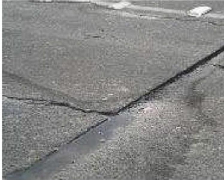
*Figure 71 Faulting Up-Close a Bus Stop*
