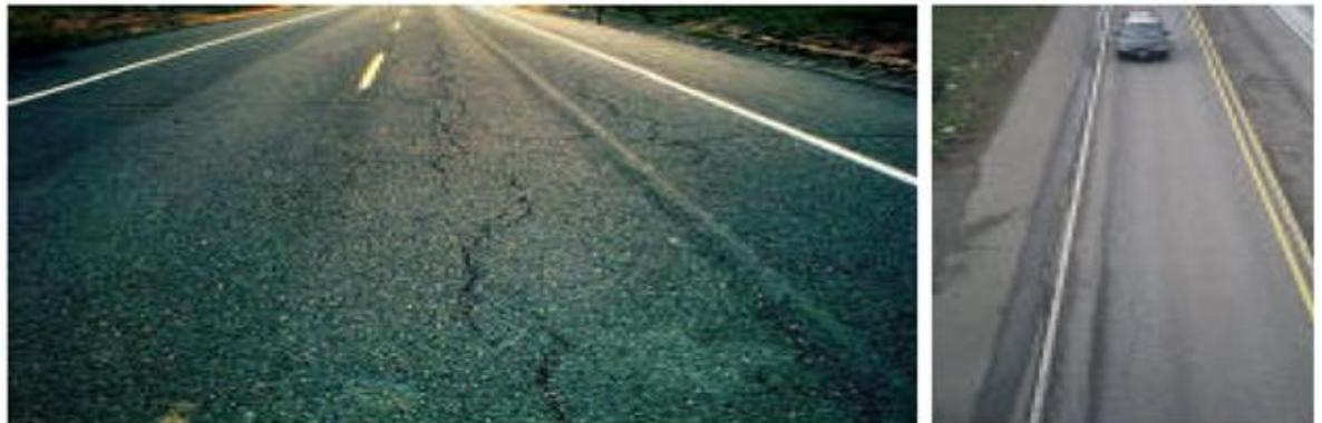
*Figure 29 Longitudinal Cracking as the Onset of Fatigue Cracking*
