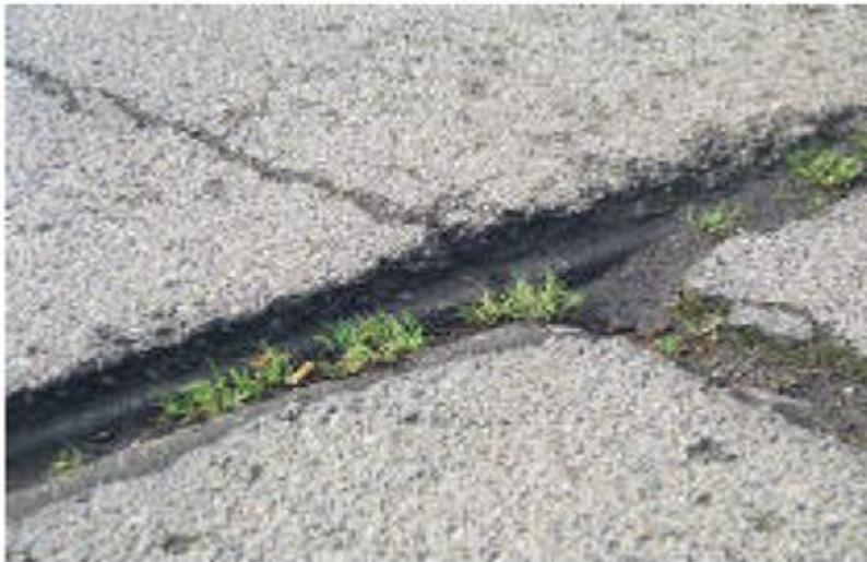
*Figure 28 Joint Reflection Cracking Close-Up*
