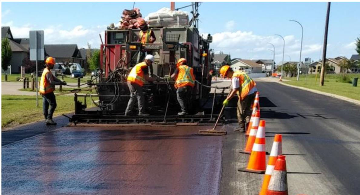
*Figure 59 Microsurfacing Application*
