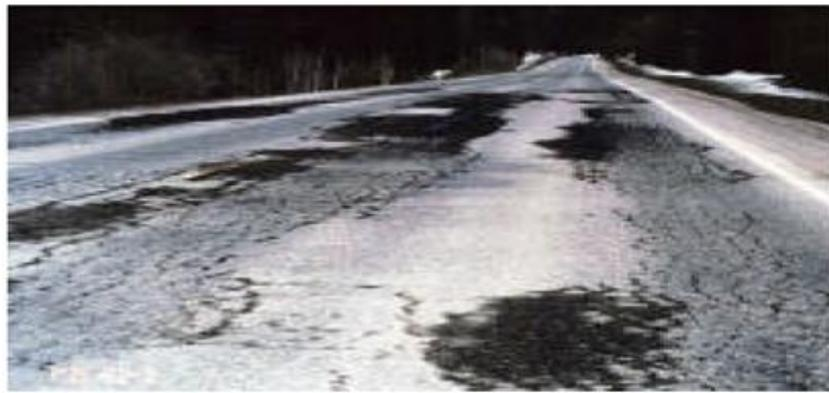
*Figure 20 Fatigue Cracking from Frost Action*
