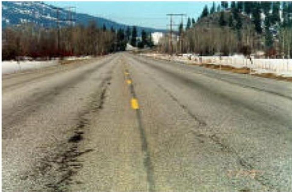
*Figure 49 Raveling Due to Low Density*
