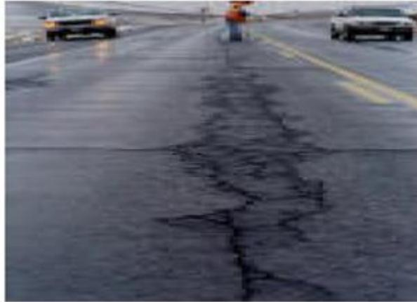
*Figure 43 Fatigue Failure from Stripping*
