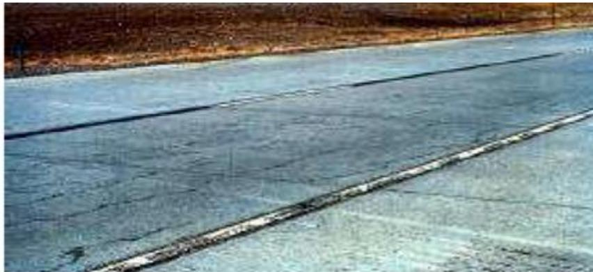
*Figure 89 Severe Shrinkage Cracking*
