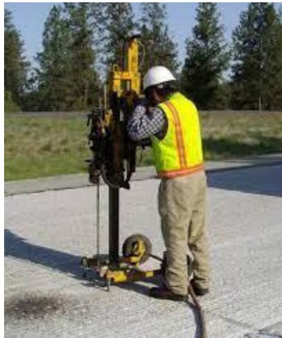
*Figure 92 Slab Stabilization*
