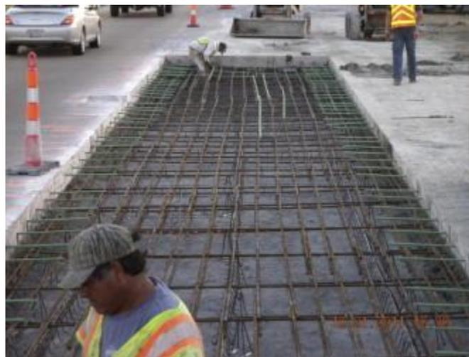
*Figure 95 Full Depth Repair*
