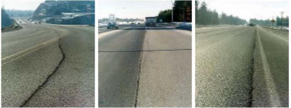
*Figure 30 Longitudinal Cracking from Poor Joint Construction*
