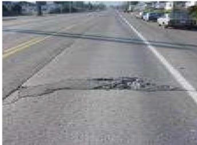
*Figure 91 Spalling from a Bad Construction Joint*
