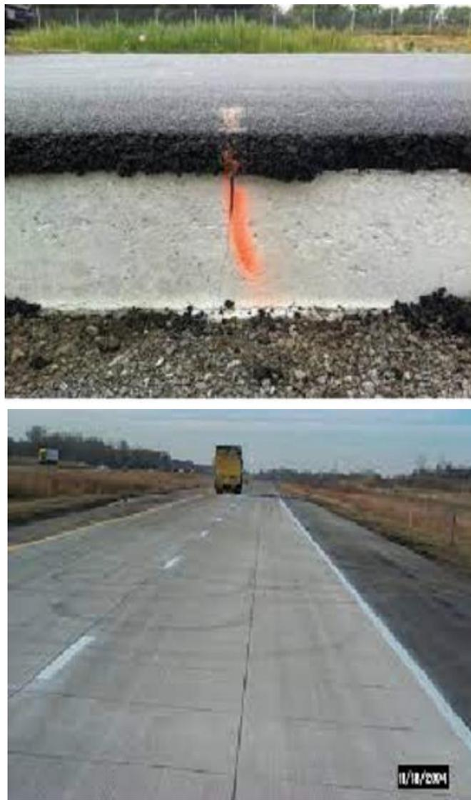
*Figure 2 Composite Pavement Black Topping (top) and White Topping (bottom)*
