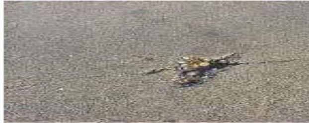
*Figure 90 Spalling*
