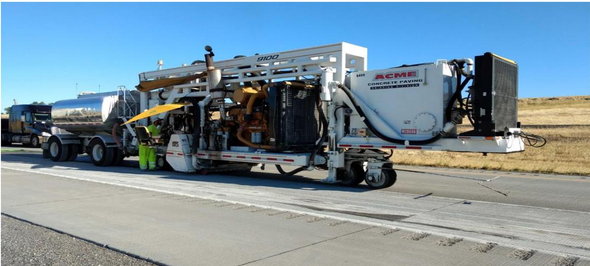
*Figure 99 Diamond Grinding*
