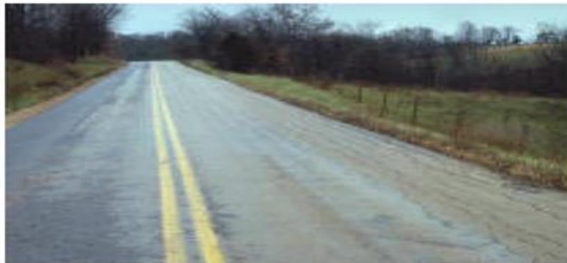
*Figure 21 Fatigue Cracking from Edge Failure*
