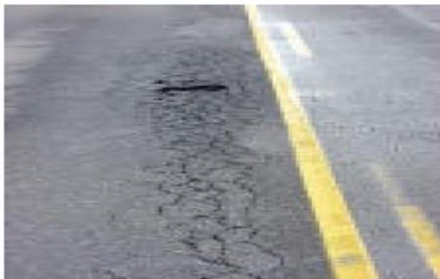
*Figure 37 Developing Pothole*
