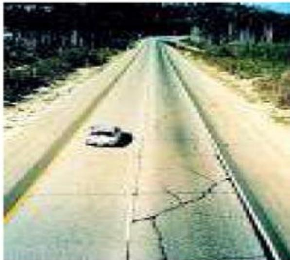
*Figure 75 Panel Cracking in the Truck Lane*
