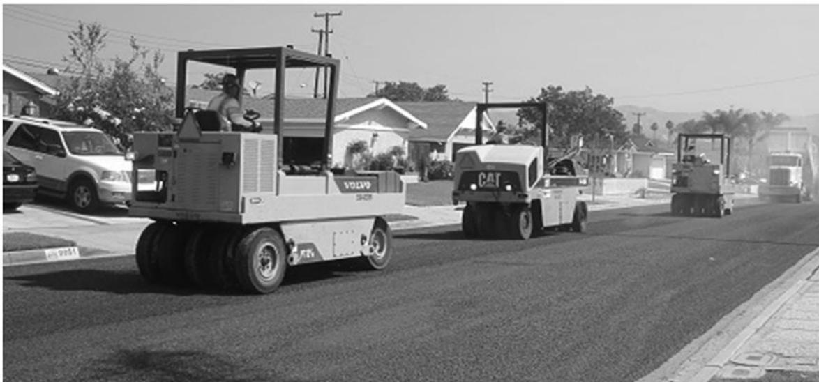
*Figure 56 Chip Seal*
