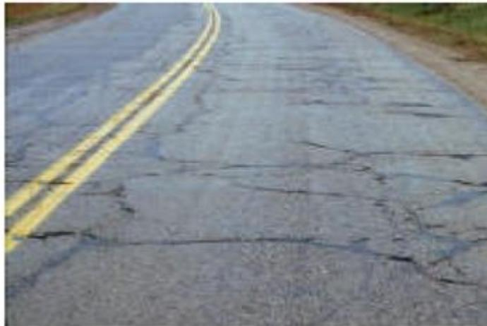
*Figure 24 Block Cracking*
