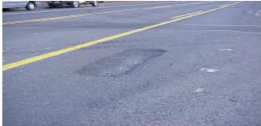
*Figure 31 Failing Patch*
