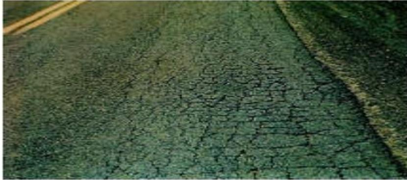
*Figure 19 Bad Fatigue Cracking*
