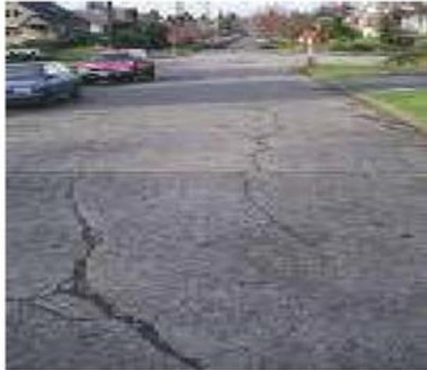
*Figure 74 Panel Crack on a Residential Street*
