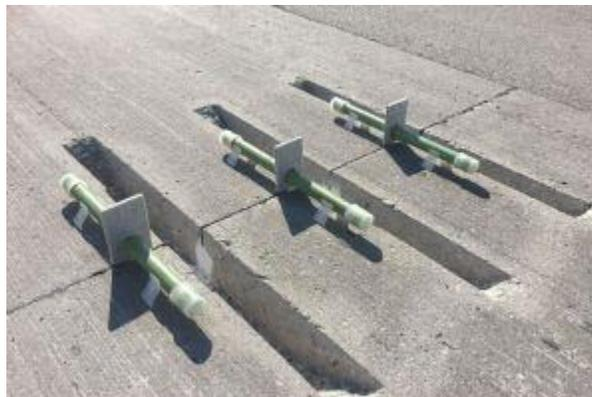
*Figure 97 Dowel Bars Retrofit*
