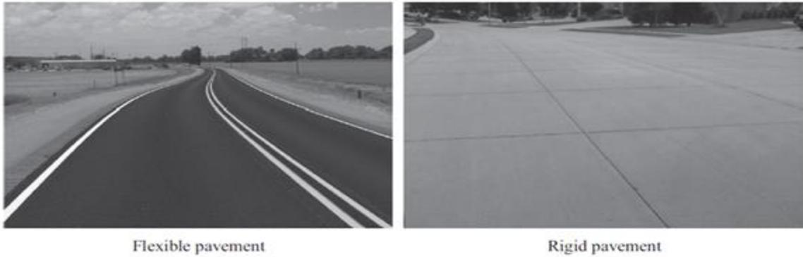
*Figure 1 Flexible and Rigid Pavements*
