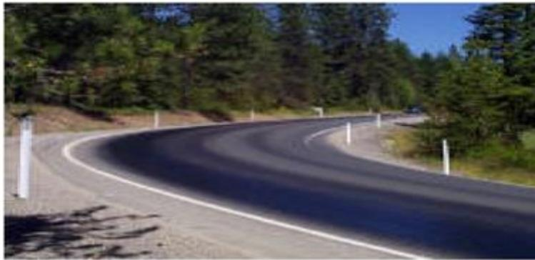
*Figure 23 HMA Bleeding from Overasphalting*
