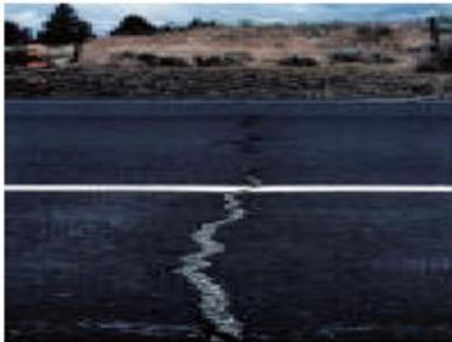
*Figure 45 Smaller Patched Thermal Crack*
