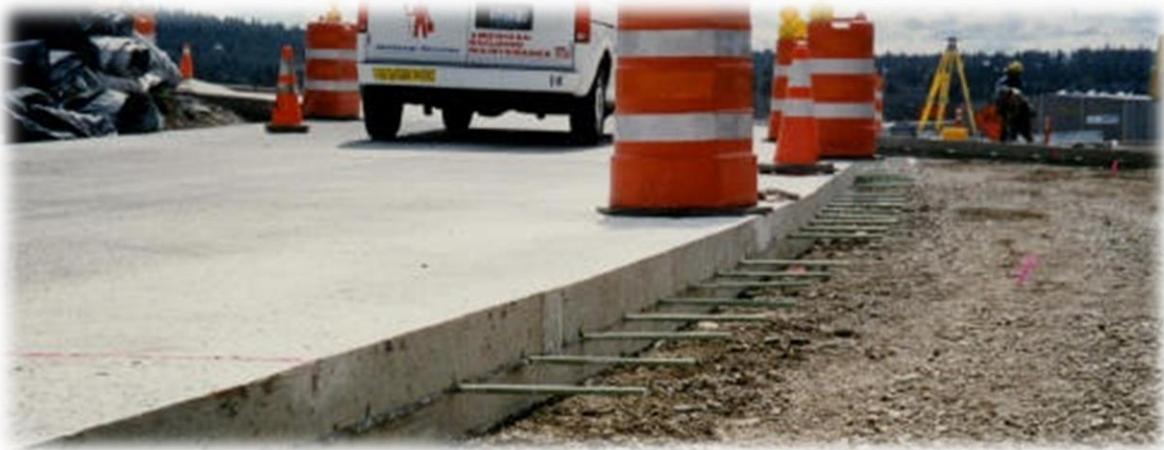
*Figure 16 Tie Bars in Rigid Pavements*
