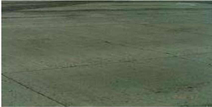
*Figure 88 Shrinkage Cracks on Brand New Slabs*
