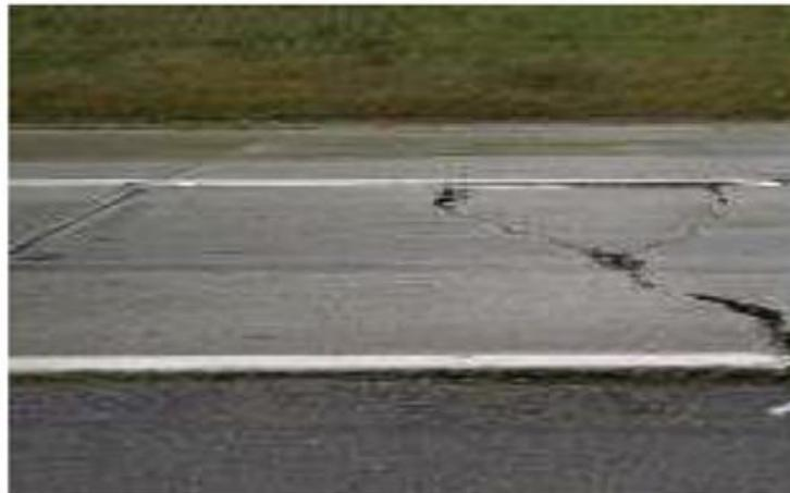
*Figure 73 Large Panel Crack*
