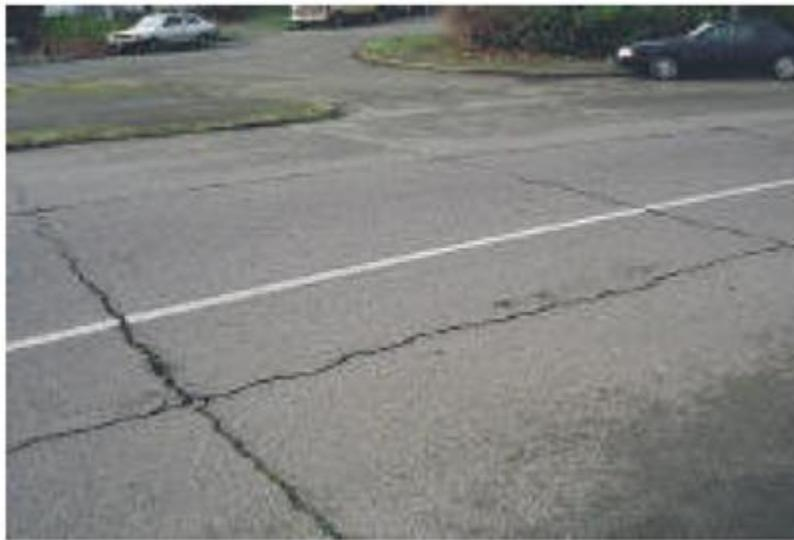
*Figure 27 Joint Reflection Cracking on an Arterial*
