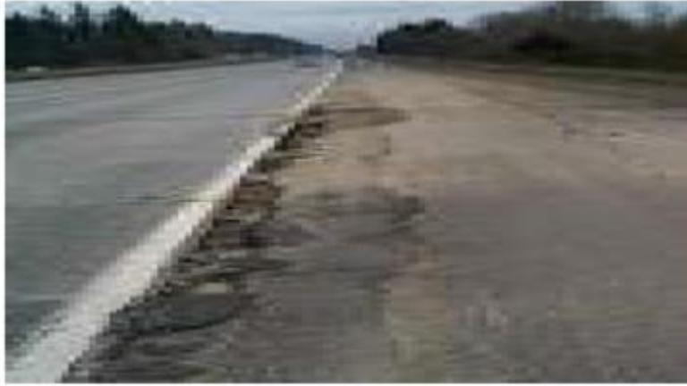
*Figure 83 Pumping Damage*
