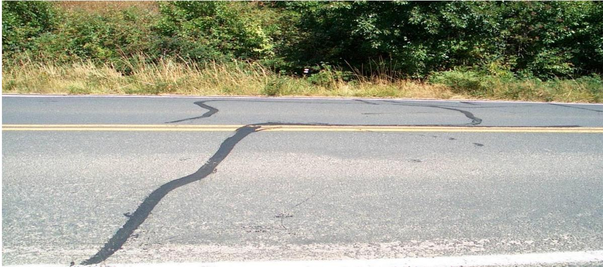
*Figure 102 Crack Sealing*
