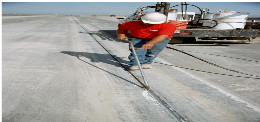
*Figure 101 Joint Resealing*
