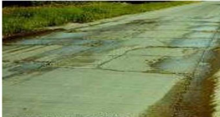
*Figure 84 Broken Slabs with Pumping Evidence*
