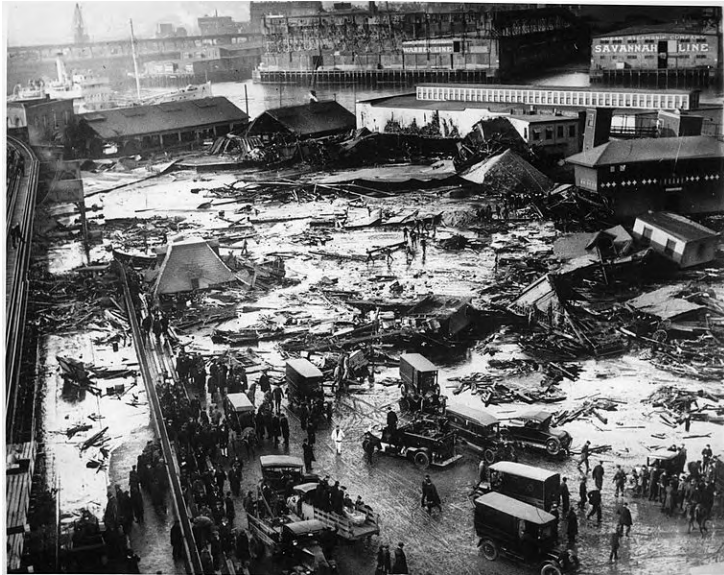
Figure 1. Aftermath of molasses tank failure
