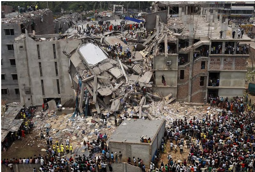
Figure 2. Aerial view of collapse.
