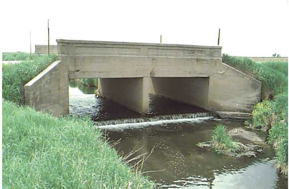
Figure P.3.1 Culvert Structure
