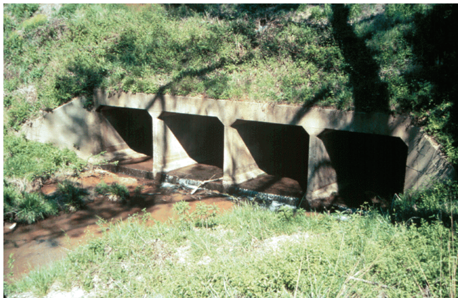
Figure P.3.10 Multiple Cell Concrete Culvert
