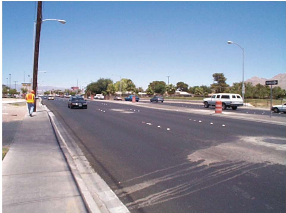
Figure P.3.26 Approach Roadway at a Culvert Site
