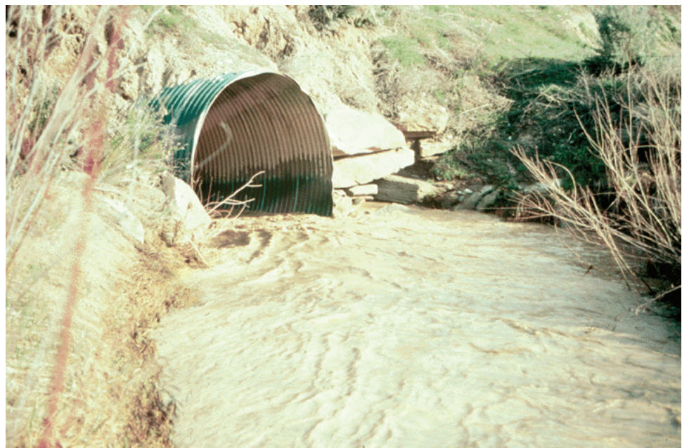
Figure P.3.15 Culvert End Projection
