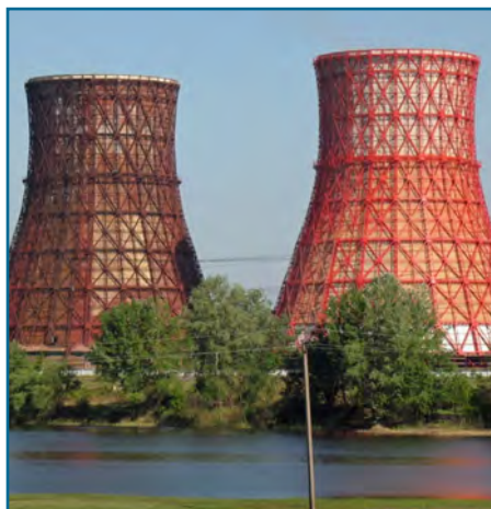
Figure 5. Hyperbolic Cooling Towers (Source: Victor Vizuz).
