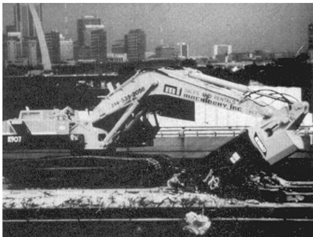
Figure 5-2. Boom-mounted concrete crusher
