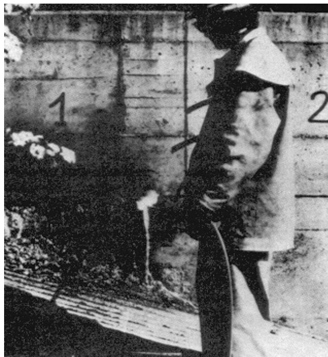
Figure 5-6. Thermal lance
