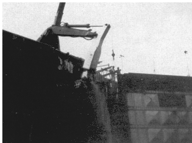
Figure 5-11. Rotary-head milling
