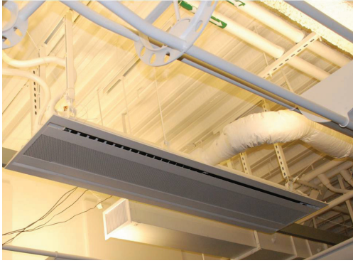
Figure 13. Chilled beams in a T-bar ceiling.
