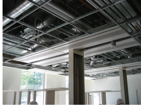
Figure 13. Chilled beams in a T-bar ceiling.
