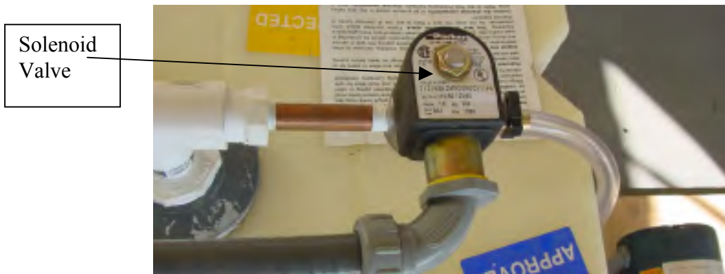
Figure 3: Normally closed solenoid valve
