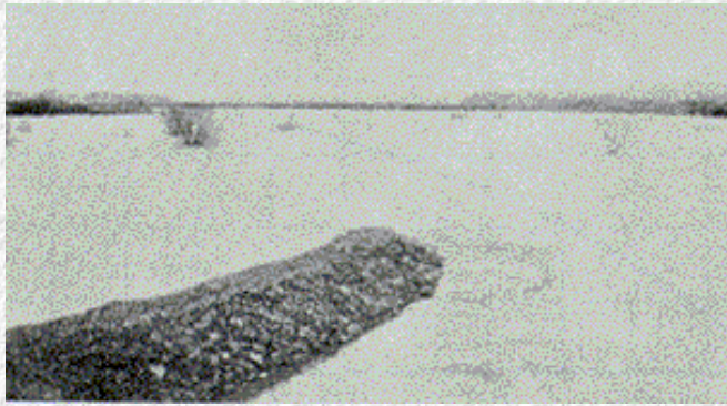
Figure 32. Spur dike on 45° skewed bridge over Susquehanna River at Nanticoke Pa.
