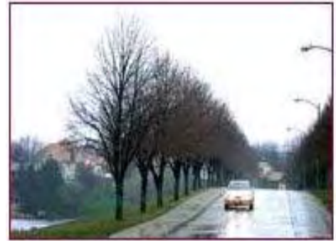
Figure 2. Example dam with problematic trees in Nebraska.
