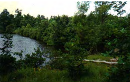
Figure 3. Example dam with inspection-hindering trees in Tennessee.
