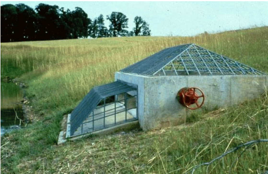
Figure 3-12 Typical Principal Spillway Outlet Structure
