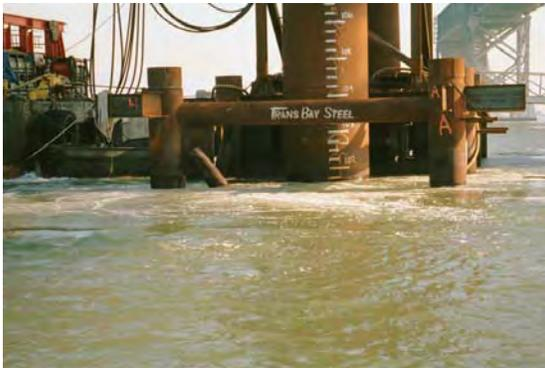
**Figure 3-9. Air bubble curtain in operation.**
