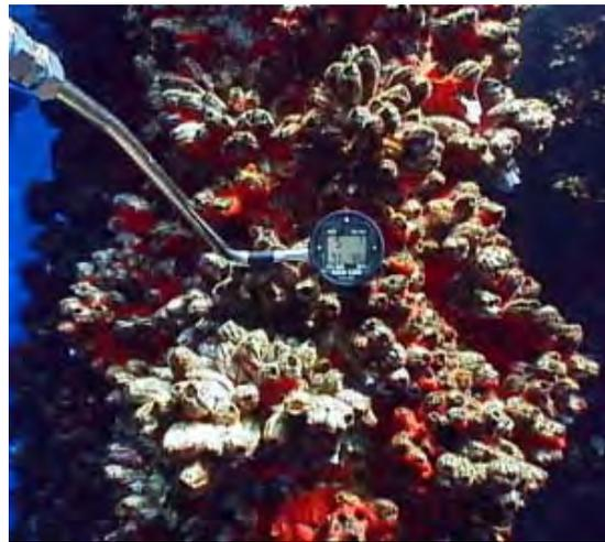
Figure 3-6. Mollusks comprise the largest portion of biomass on many offshore platforms. Source: MMS, [http://www.gomr.mms.gov/homepg/regulate/envIRON/studies/turning\\_to\\_the\\_sea](http://www.gomr.mms.gov/homepg/regulate/envIRON/studies/turning_to_the_sea).
