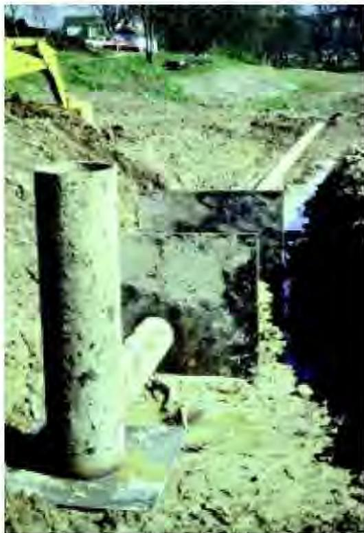
**Figure 23** Drop-inlet pipe spillways
