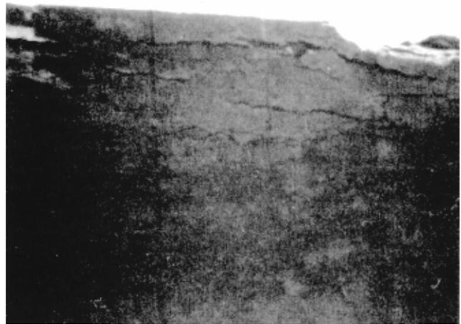
**Figure 2-10. Parallel individual cracking caused by freezing and thawing**
