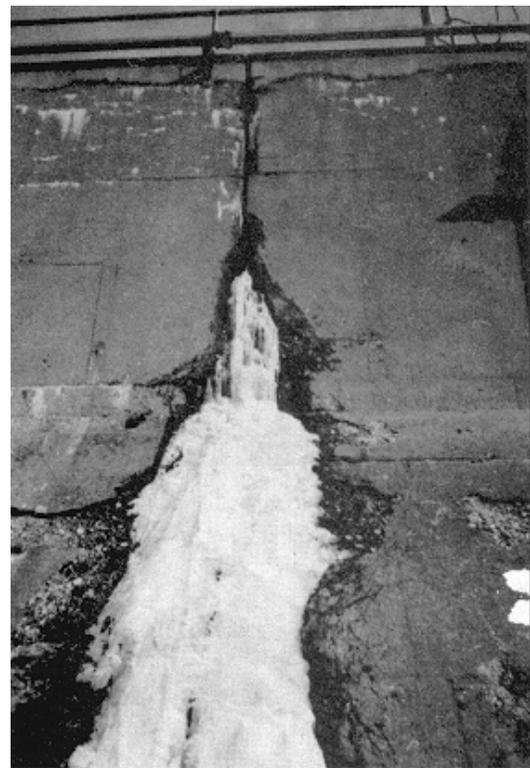
Figure 2-28. Water seepage through joint
