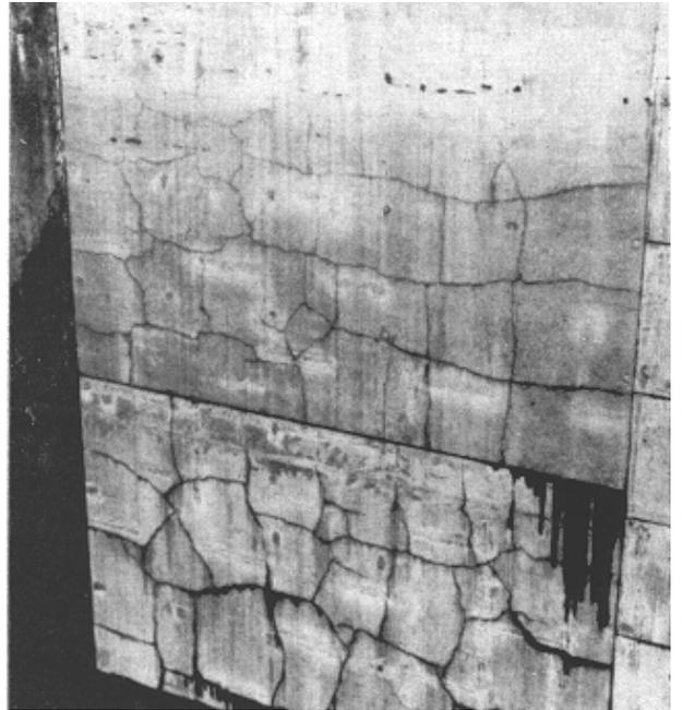
Figure 2-5. Pattern cracking caused by restrained volume changes
