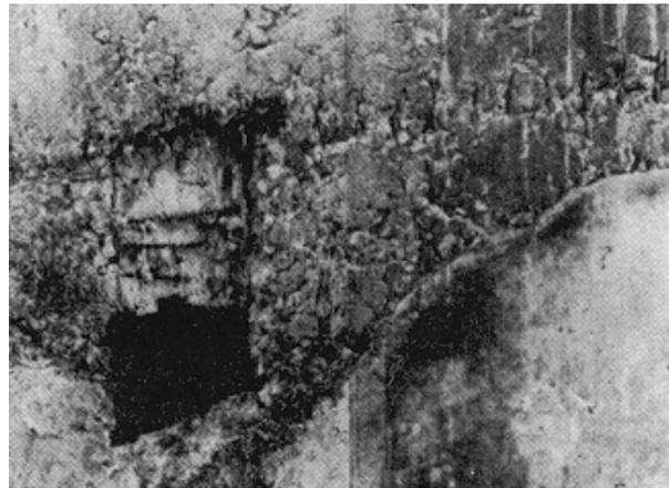
**Figure 2-2.** Honeycombing and cold joint
