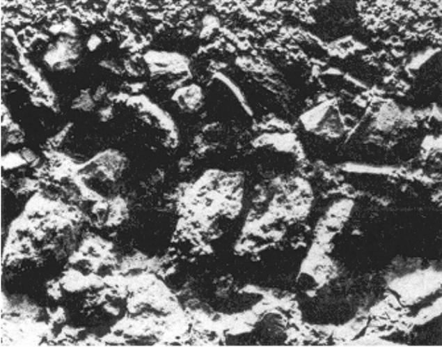
**Figure 2-21. Rough, pitted concrete surface caused by cavitation**
