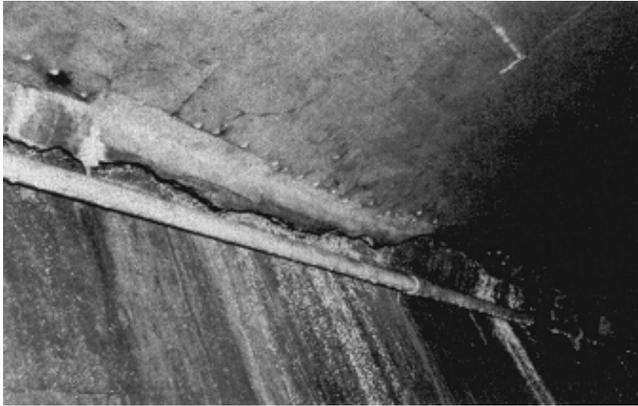
**Figure 2-11. Isolated crack caused by structural overload**
