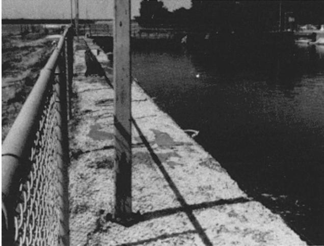
Figure 2-18. Severe scaling
