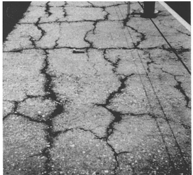
Figure 2-6. Pattern cracking resulting from alkali-silica reaction
