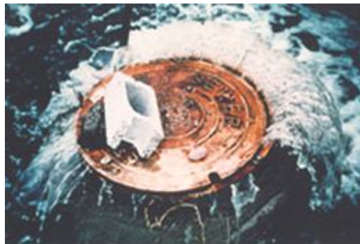
During large storm events sanitary sewers receive storm water runoff in addition to wastewater, causing them to overflow (Source: USEPA, 2000)
