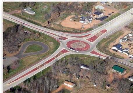
Figure 2: Roundabout with OSOW features.
