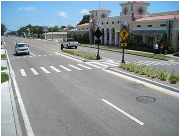
The use of curb extensions or bulb-outs should be considered to reduce the crossing distance for pedestrians. The reduction in distance reduces the time in the crossing and causes a roadway width constriction resulting in lower speeds which increases pedestrian safety.
